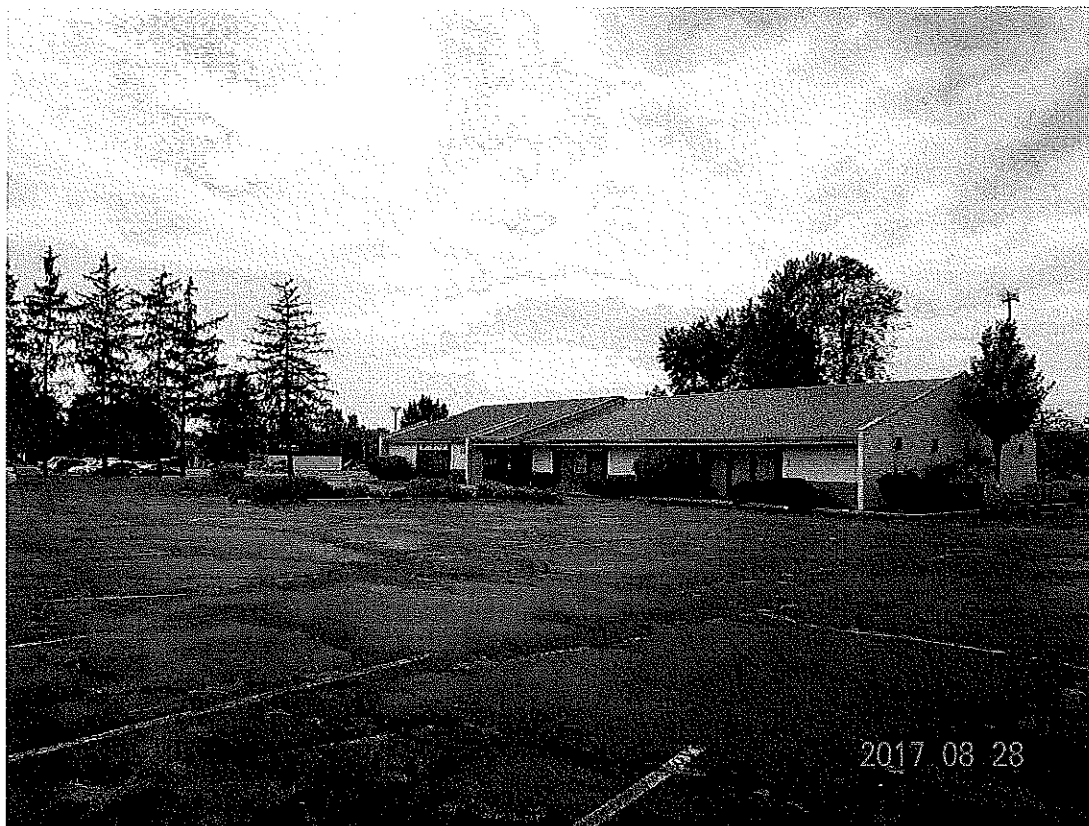
P1. Looking southwesterly toward the existing vacant commercial building on the site.
