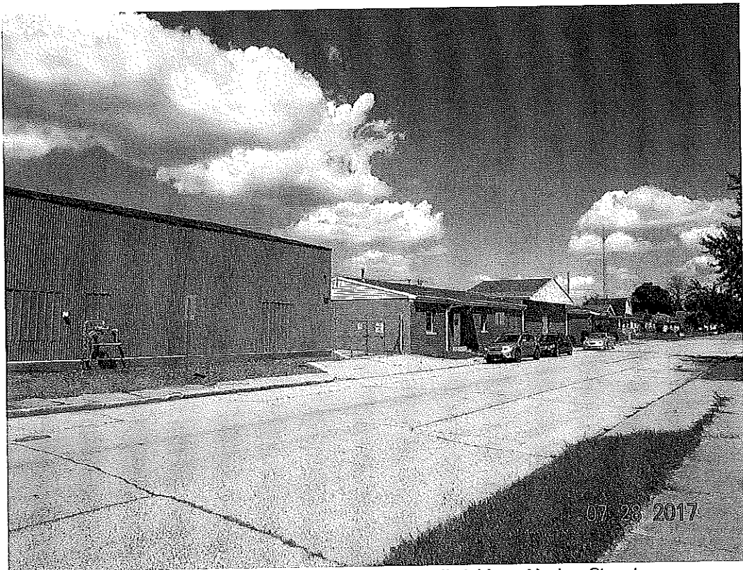
P1: Storage building (gray) and office (brick) on Marion Street
