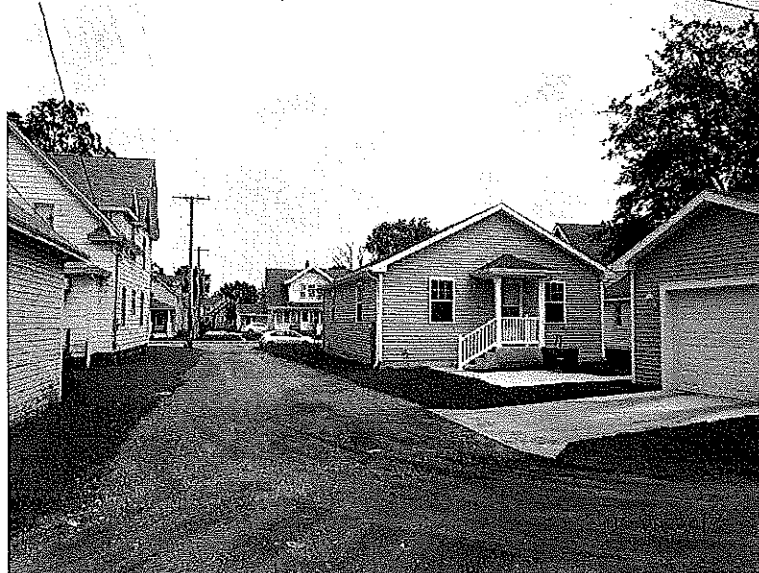
A view south of the alley to be vacated from the east-west alley
