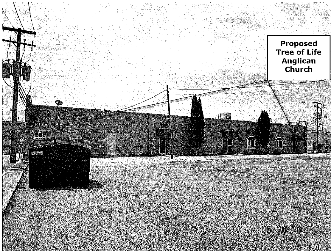
P1. Looking southwesterly toward the vacant tenant space and adjacent parking area to be used for the church.
