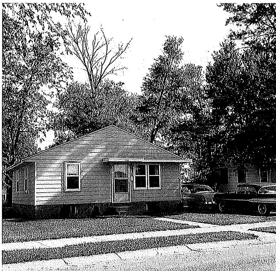
Two-Bedroom with basement: Bastogne (Photo Credit: Ruth Pavich)
