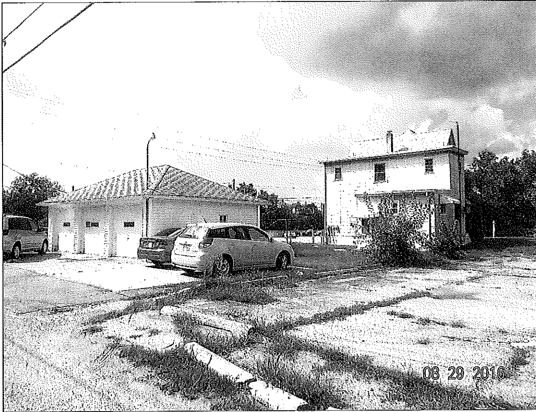
View of 1217 Lincolnway West from alley
