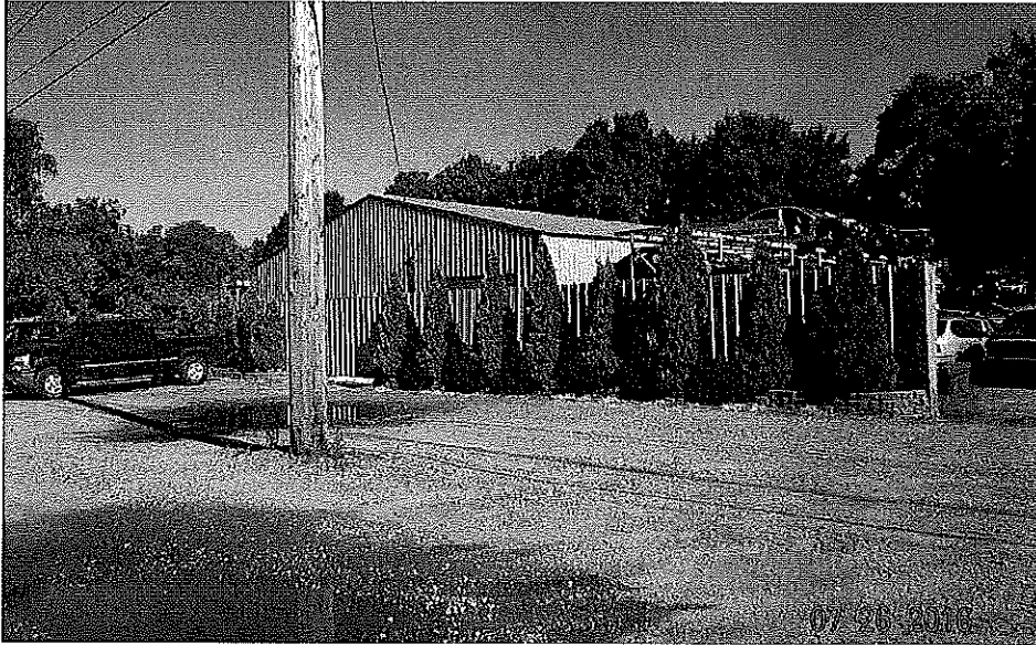
A VIEW OF THE BUILDING AT 1718 E MCKINLEY
