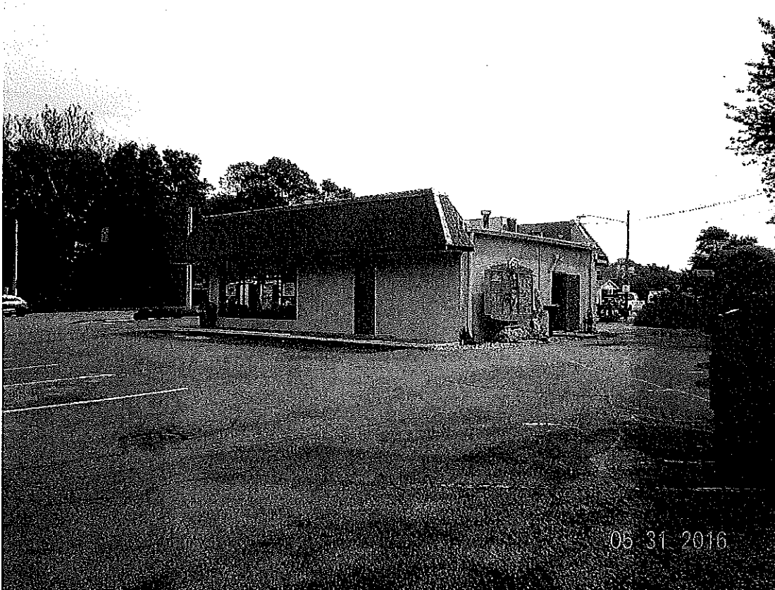
P2. Looking northeasterly into the current Dairy Queen site proposed to be redeveloped.
