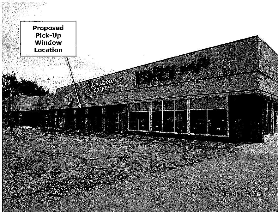
P3. Looking northeasterly from the access along River Avenue toward the proposed location for the drive-thru pick-up window.
