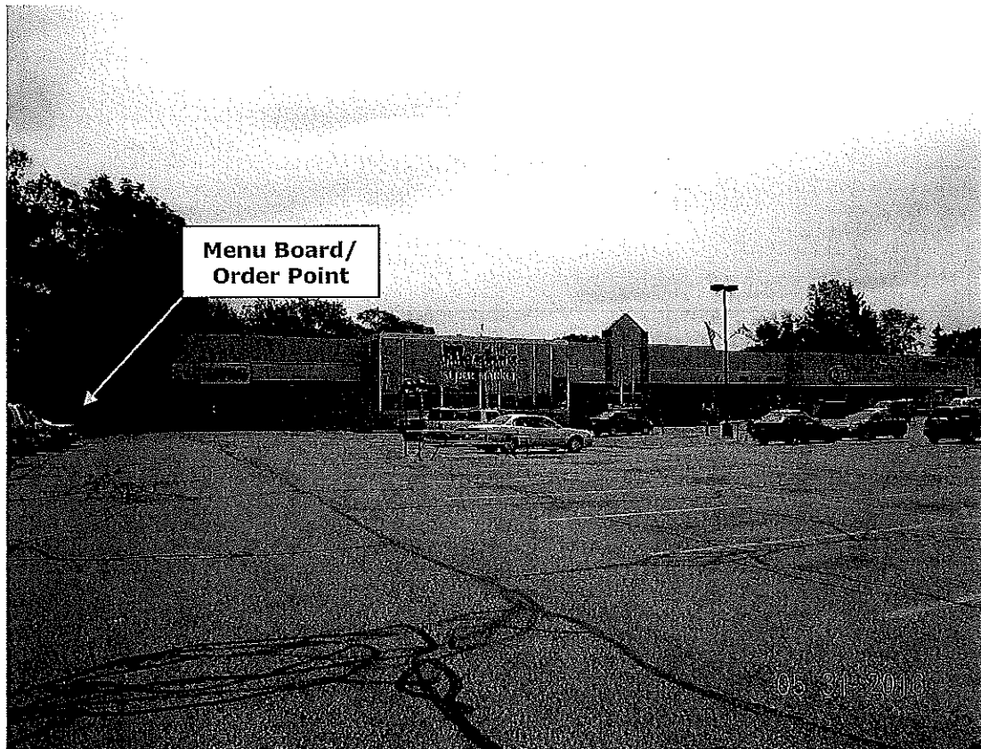
P1. Looking easterly into site and along the access drive for the proposed drive-thru.
