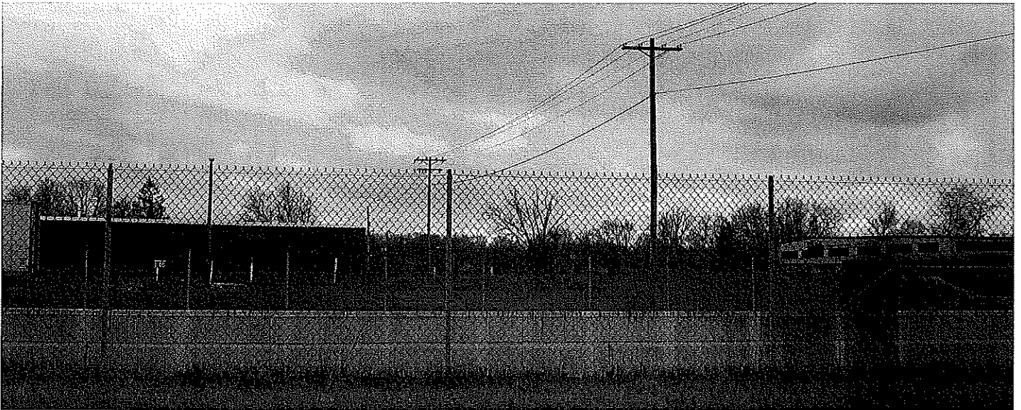
A view south at the area to be vacated
