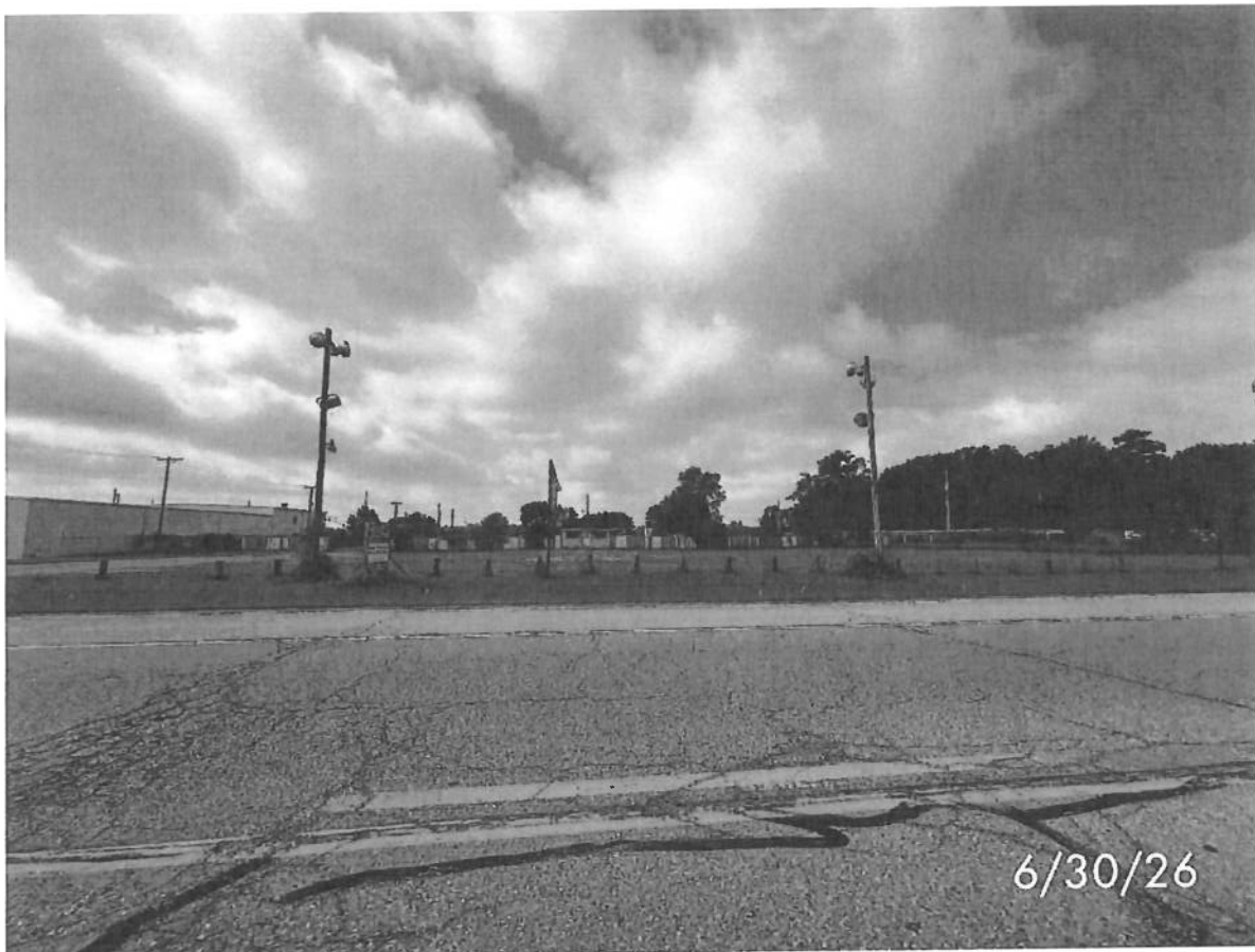
P6. Looking southerly from Lincolnway East toward the property.
