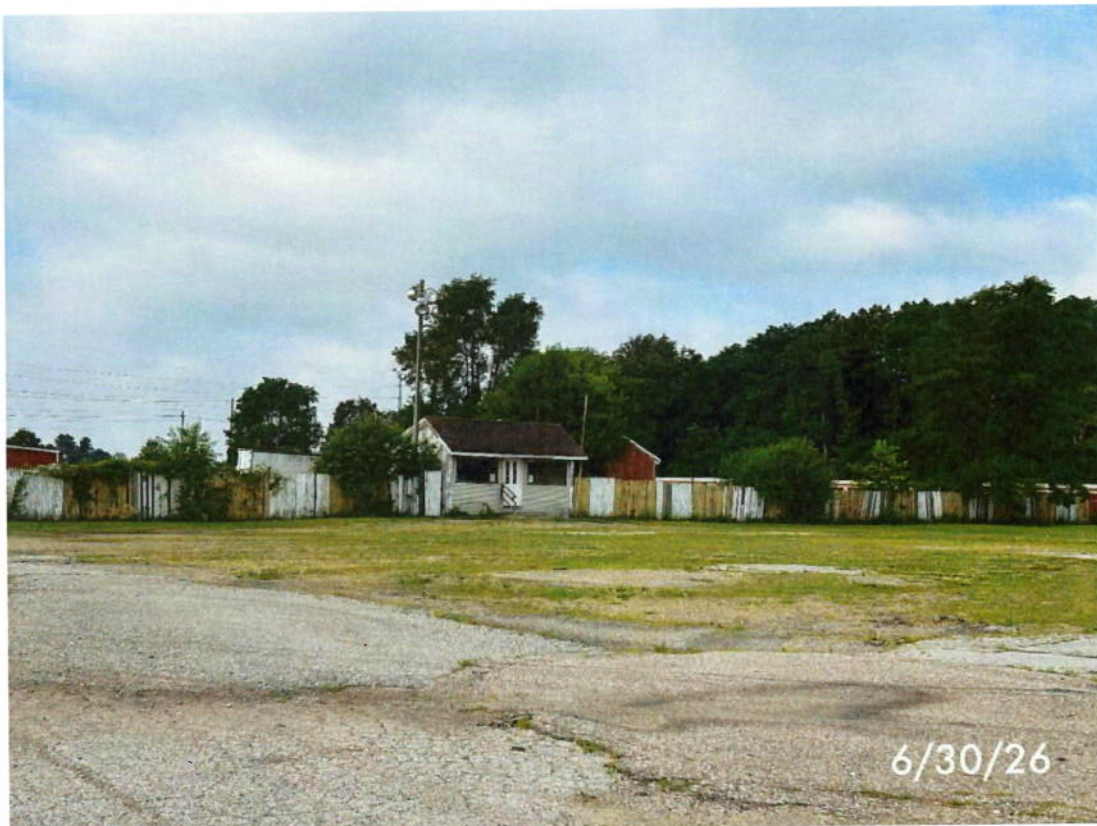
Looking southwesterly from east property line within property toward rear fence-in area.
