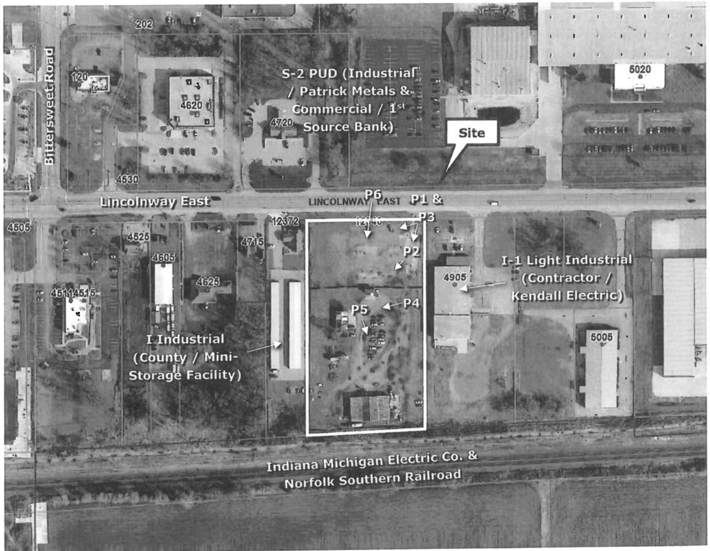
Aerial Photograph – 12340 Lincolnway East Proposed Industrial / Flex Space & Commercial Buildings
