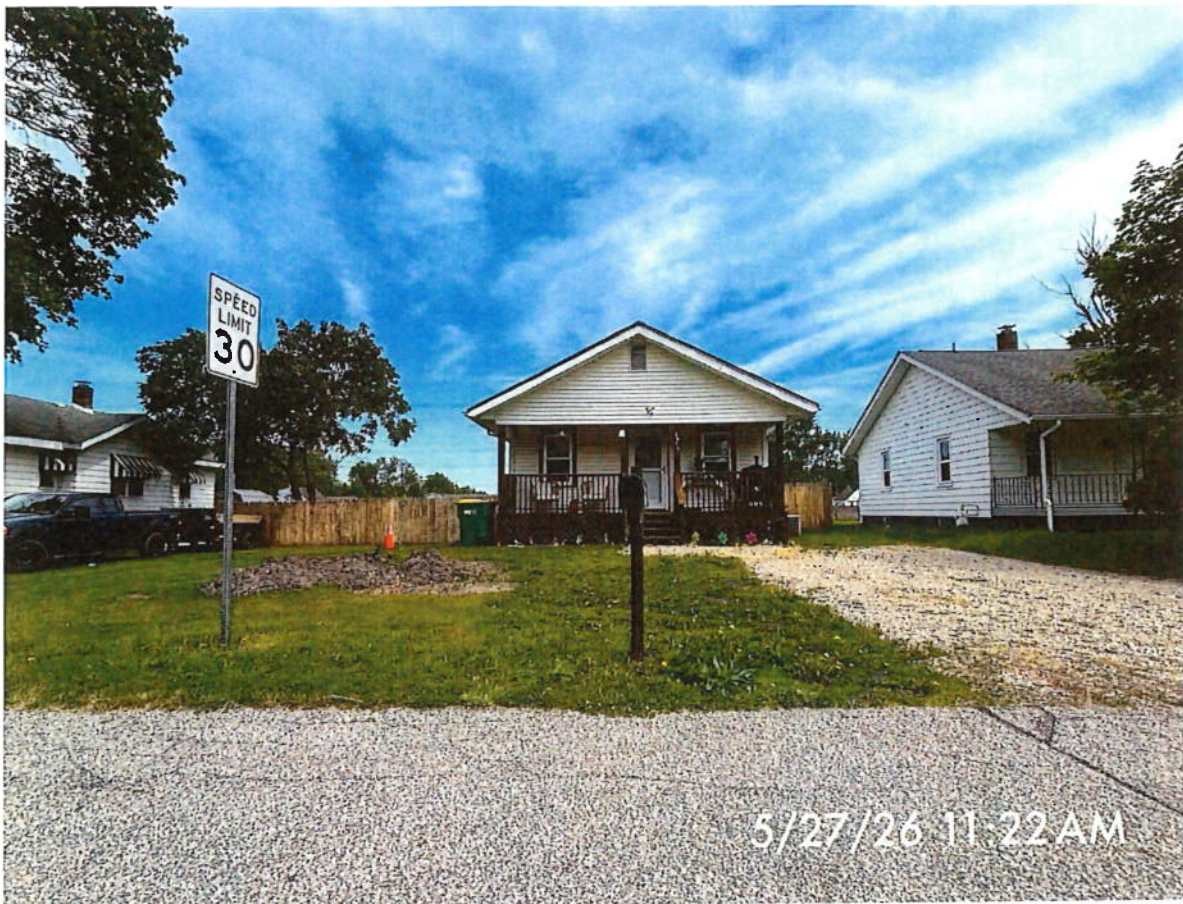
North facing from York Street
