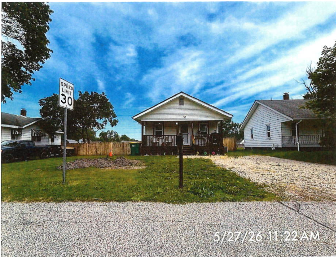
North facing from York Street
