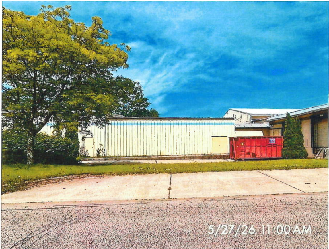
P3. Looking west from N. Cedar at the Loading Dock area
