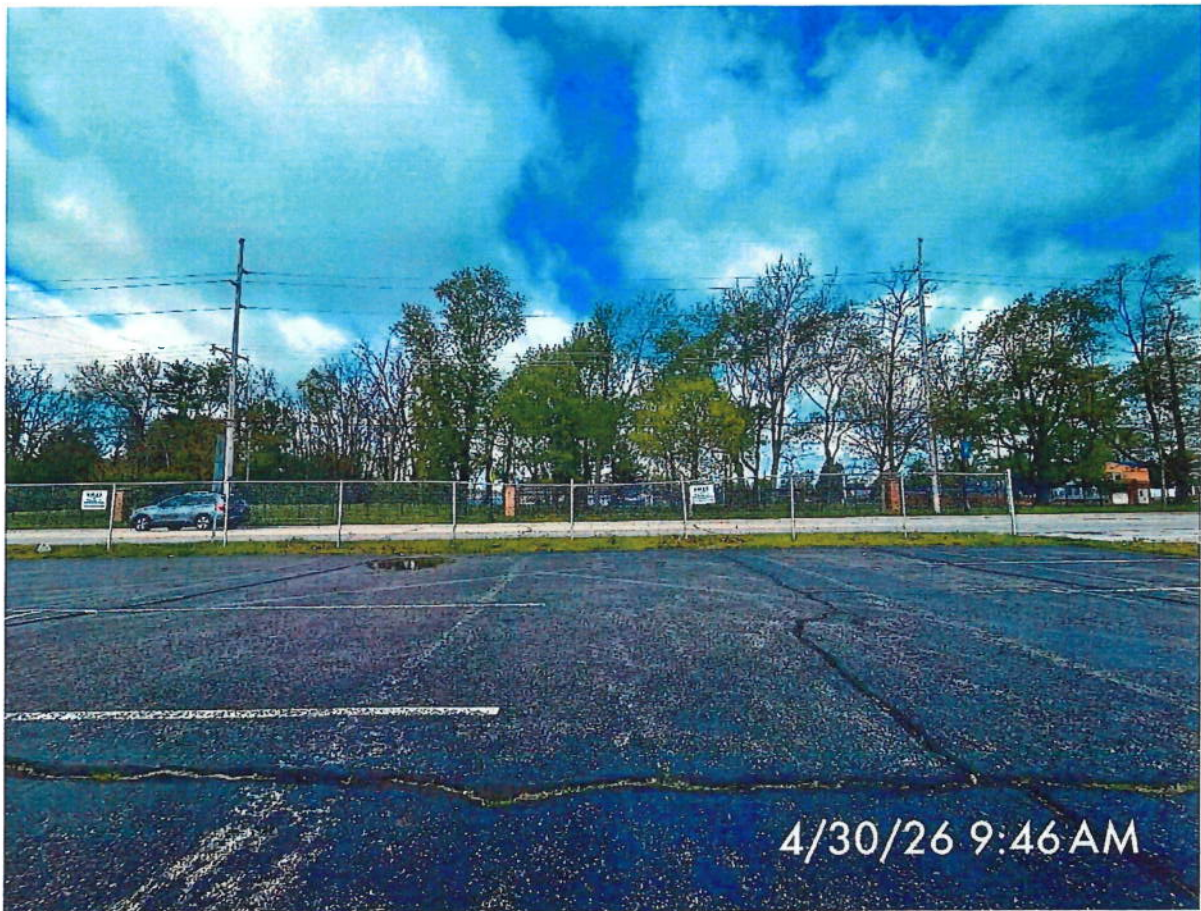
West facing from the parking lot
