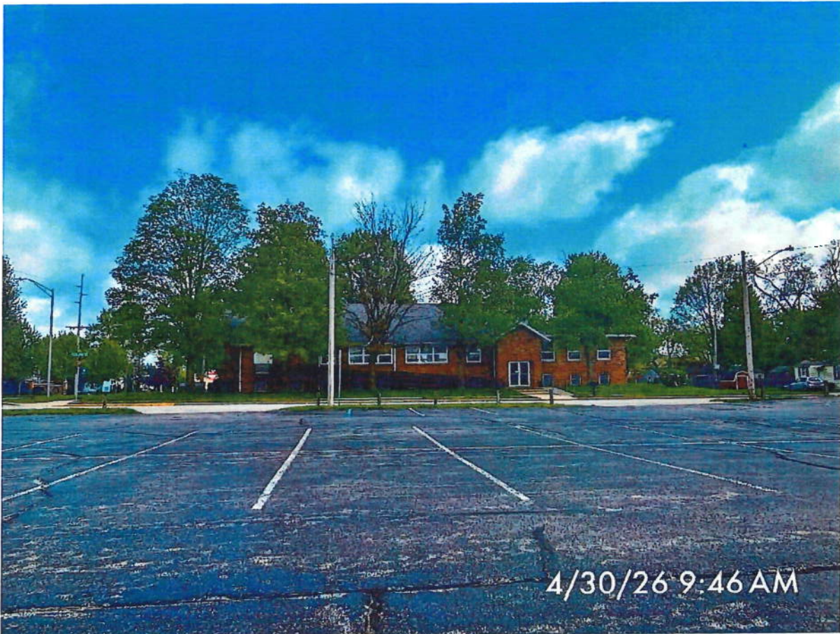
North facing from the parking lot.
