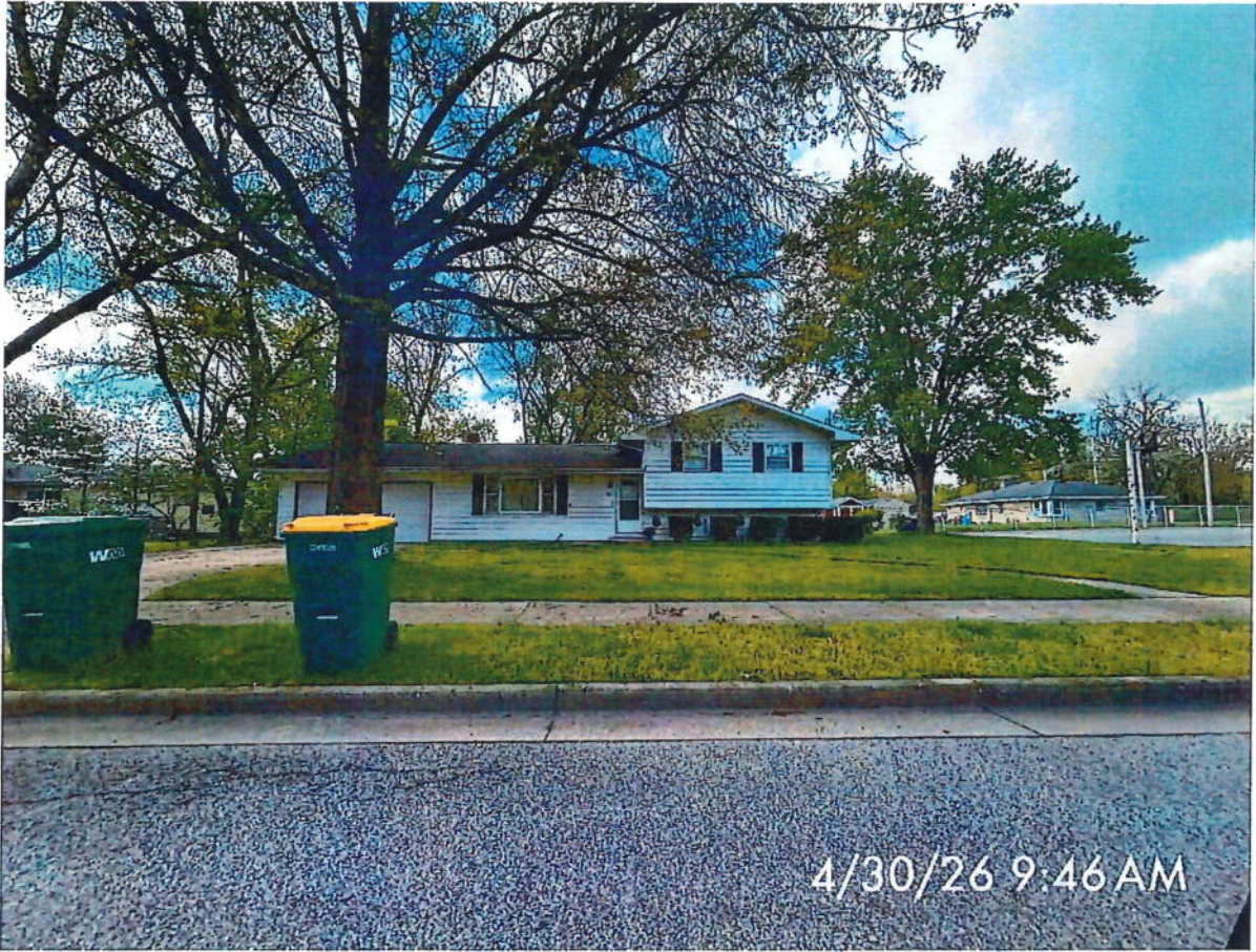
South facing from West Colfax Avenue
