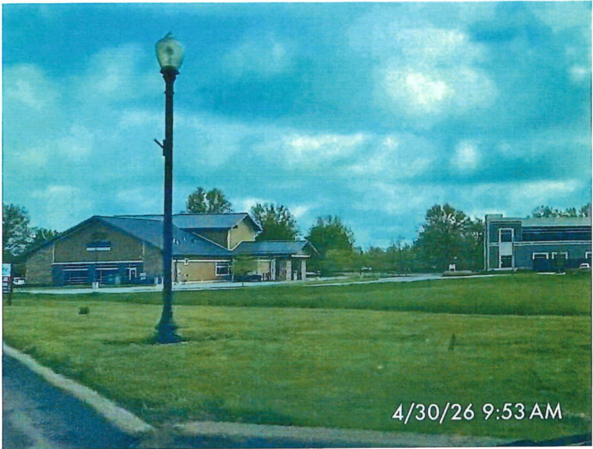
A view north along Main Street
