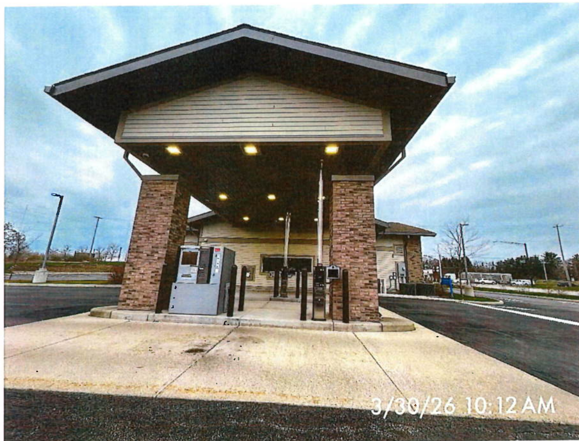
3. West facing from the parking lot
