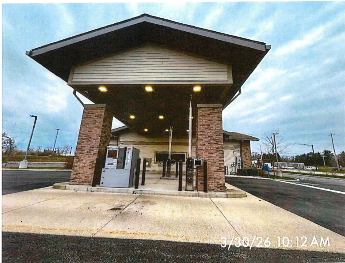
3. West facing from the parking lot
