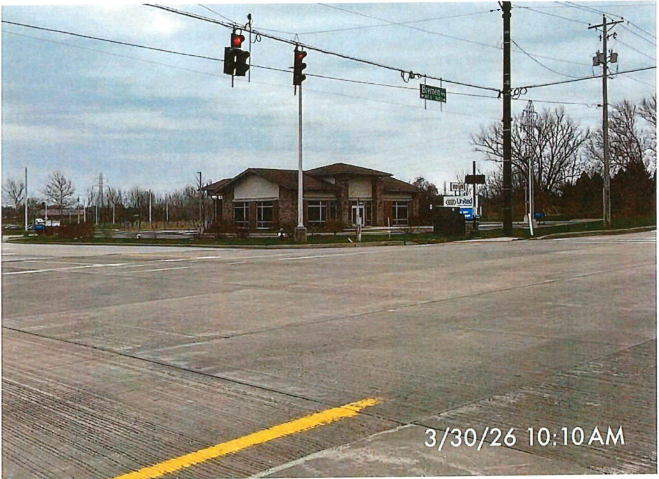
0. Southeast facing from Bremen Highway
