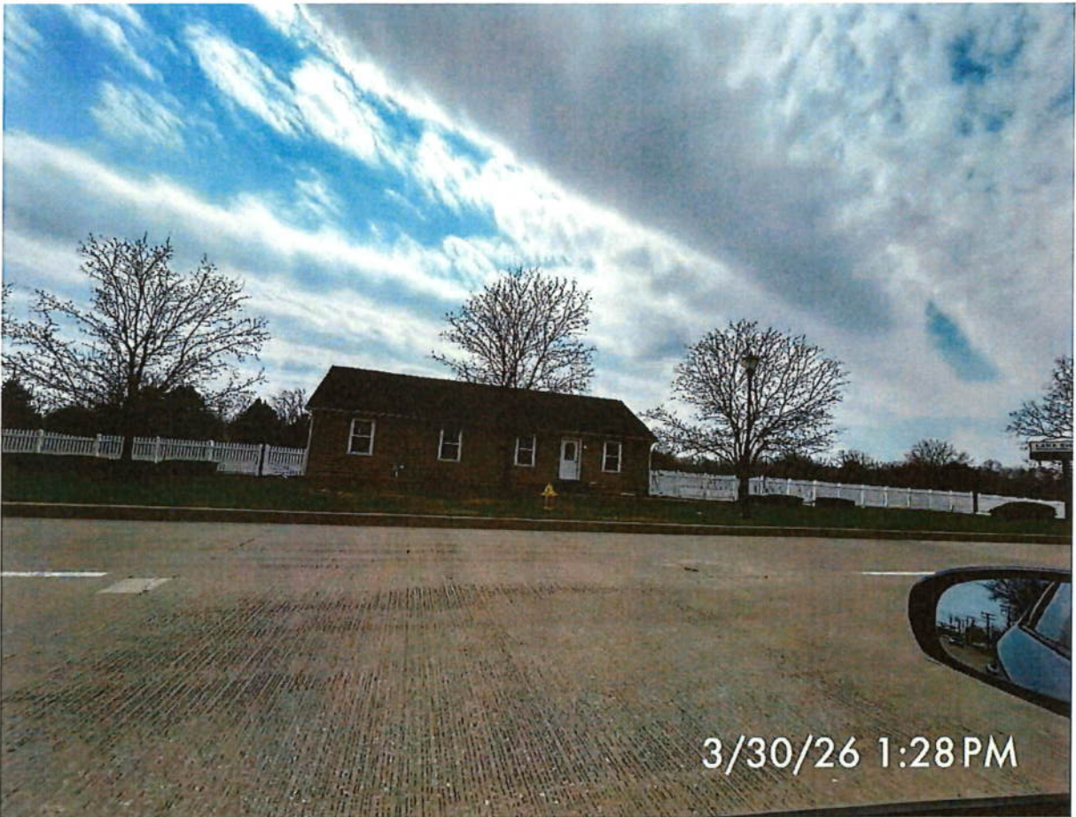
P2. Looking southerly from W. Douglas Road toward the existing office building.
