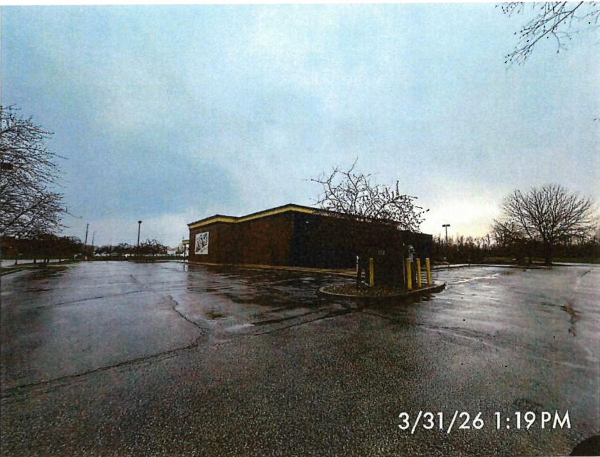
P2. Looking northwesterly toward the building from the southeast corner of the property.
