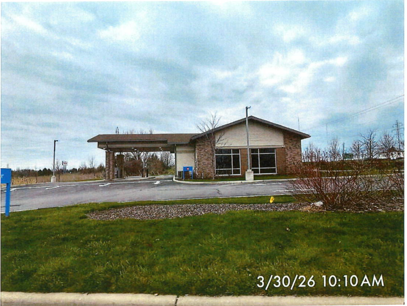
4. South facing from the parking lot
