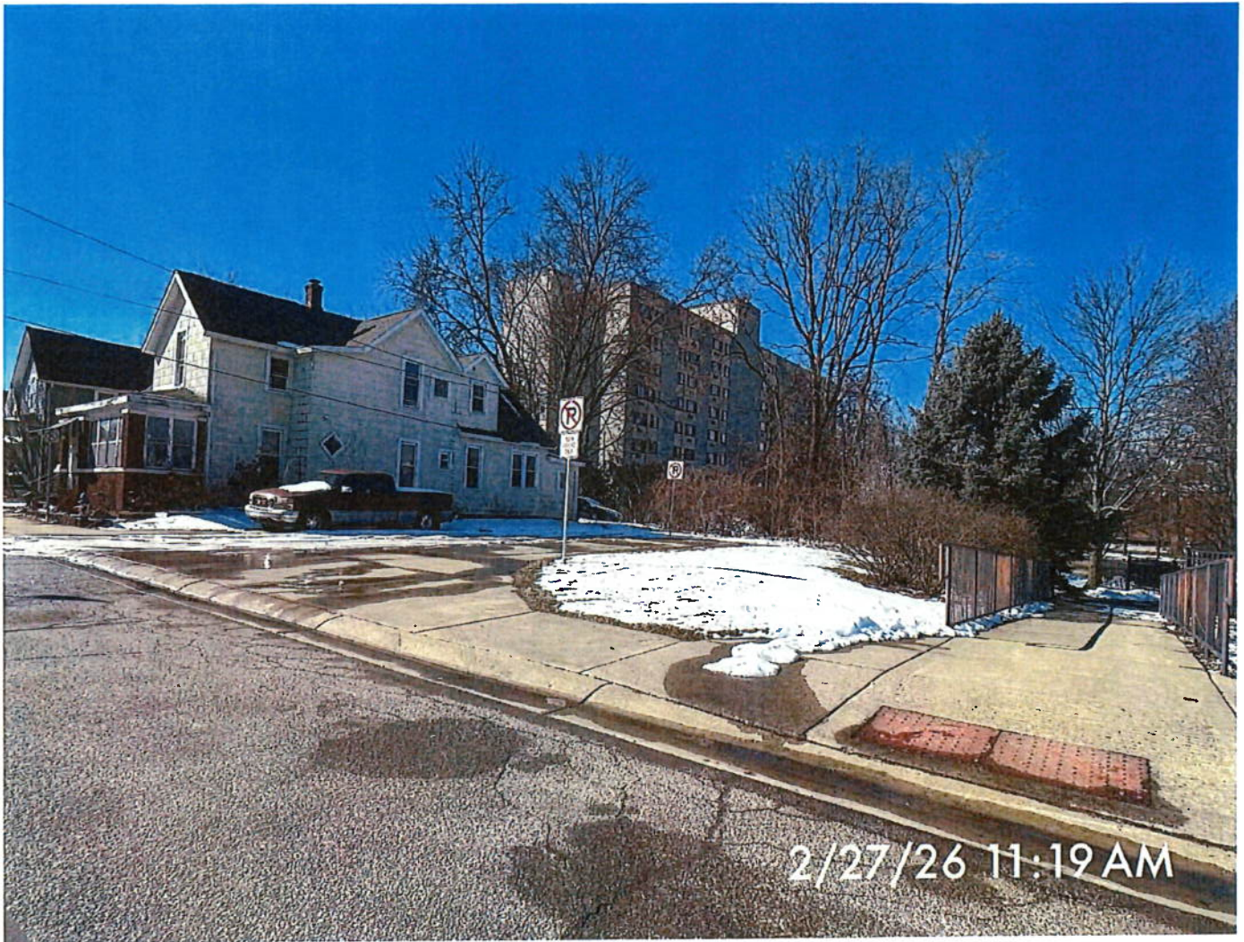
Looking south from the terminus of Towle Ave Pedestrian walkway and paved turnaround will not be affected
