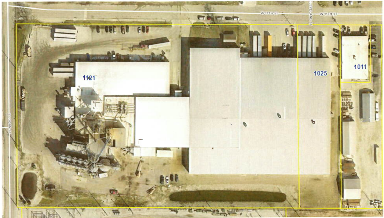
Aerial Photos of Parcels (Equipment planned to be installed in parcels labeled 1121 & 1025)
