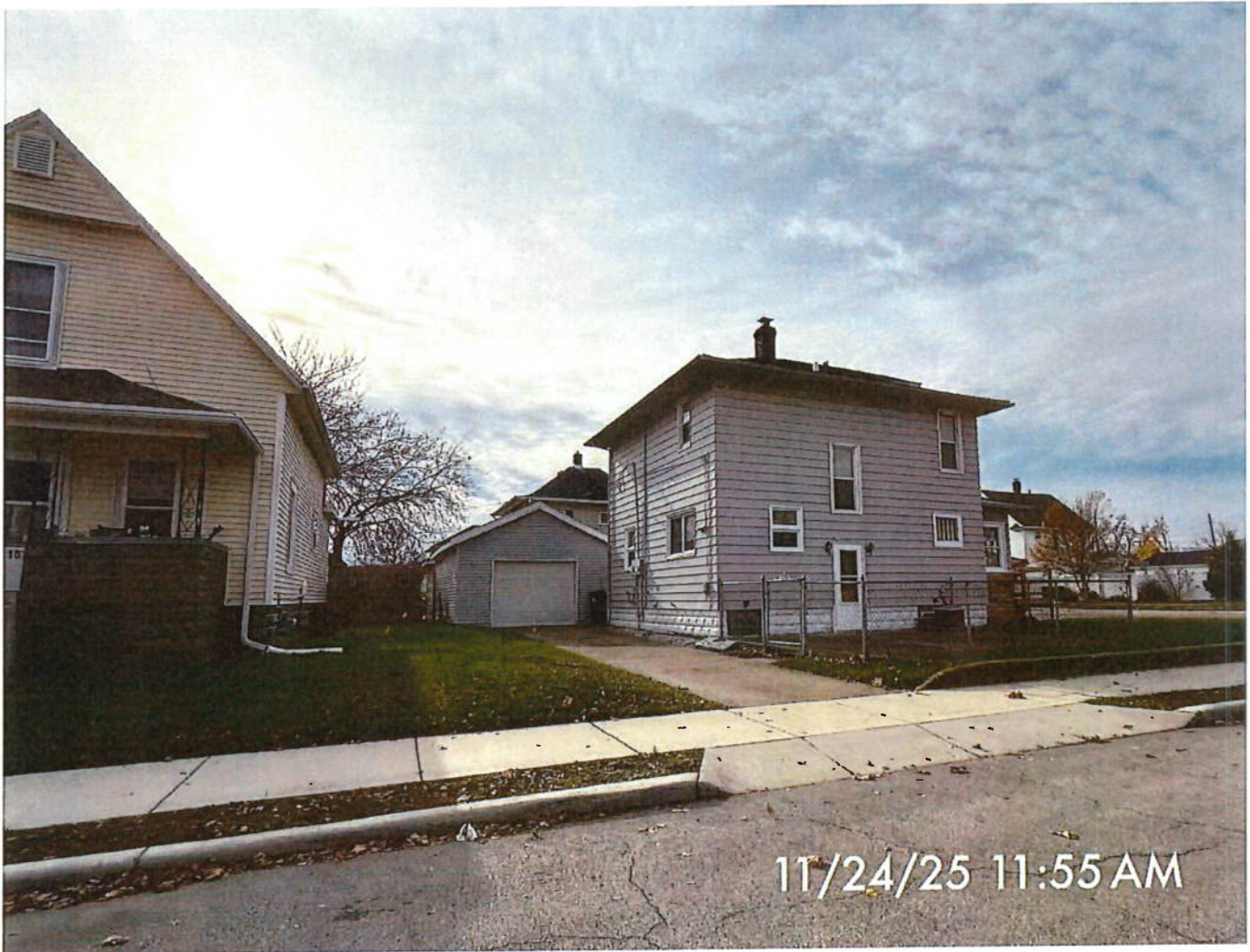
P3. A view of the garage and driveway
