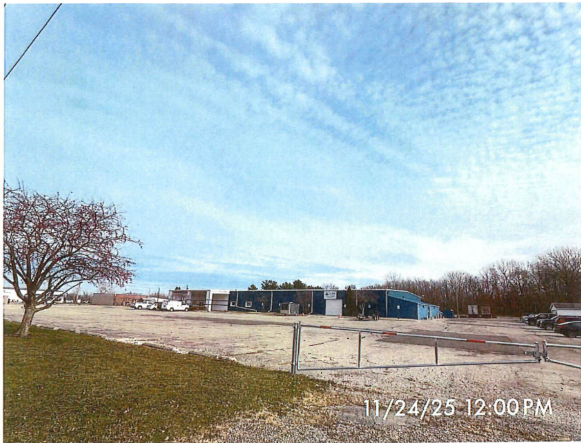
1. Northeast facing from Commonwealth Drive
