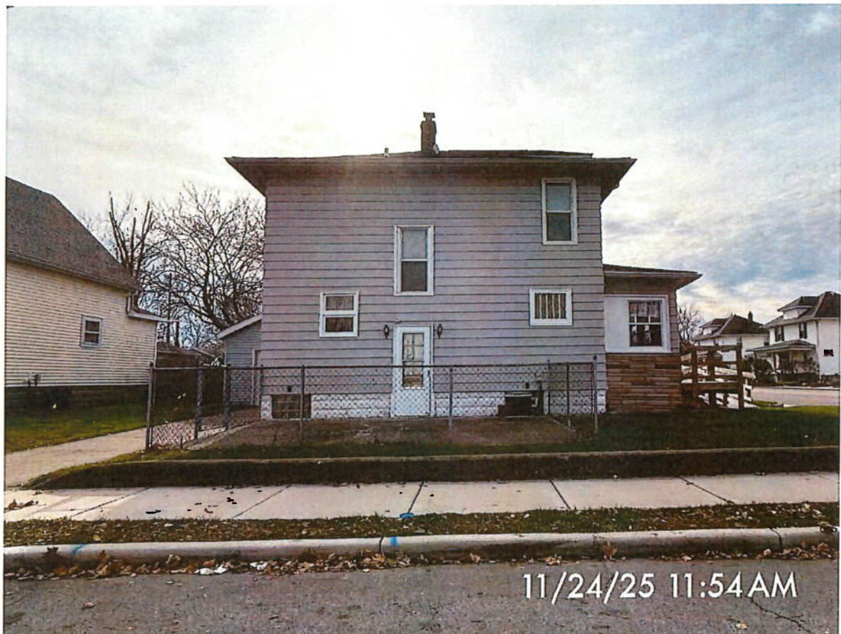
P2. A view south from East Tenth Street
