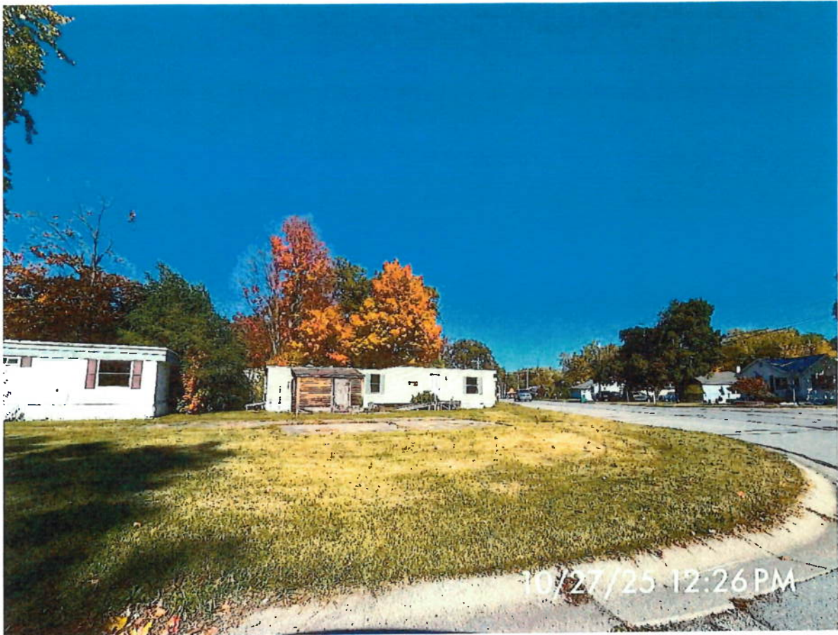
P7. Looking northerly from E. LaSalle Ave. & N. Byrkit Ave. toward the SE corner of the property.
