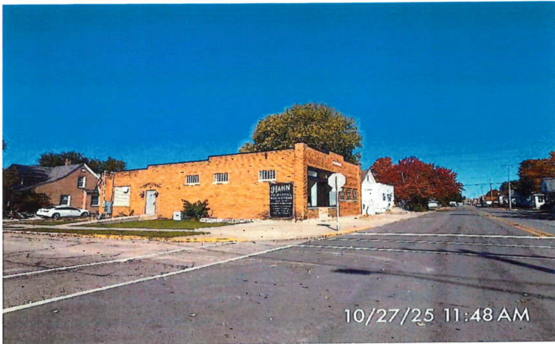
A view of the building looking northwest from intersection of Spring and W Thirteenth
