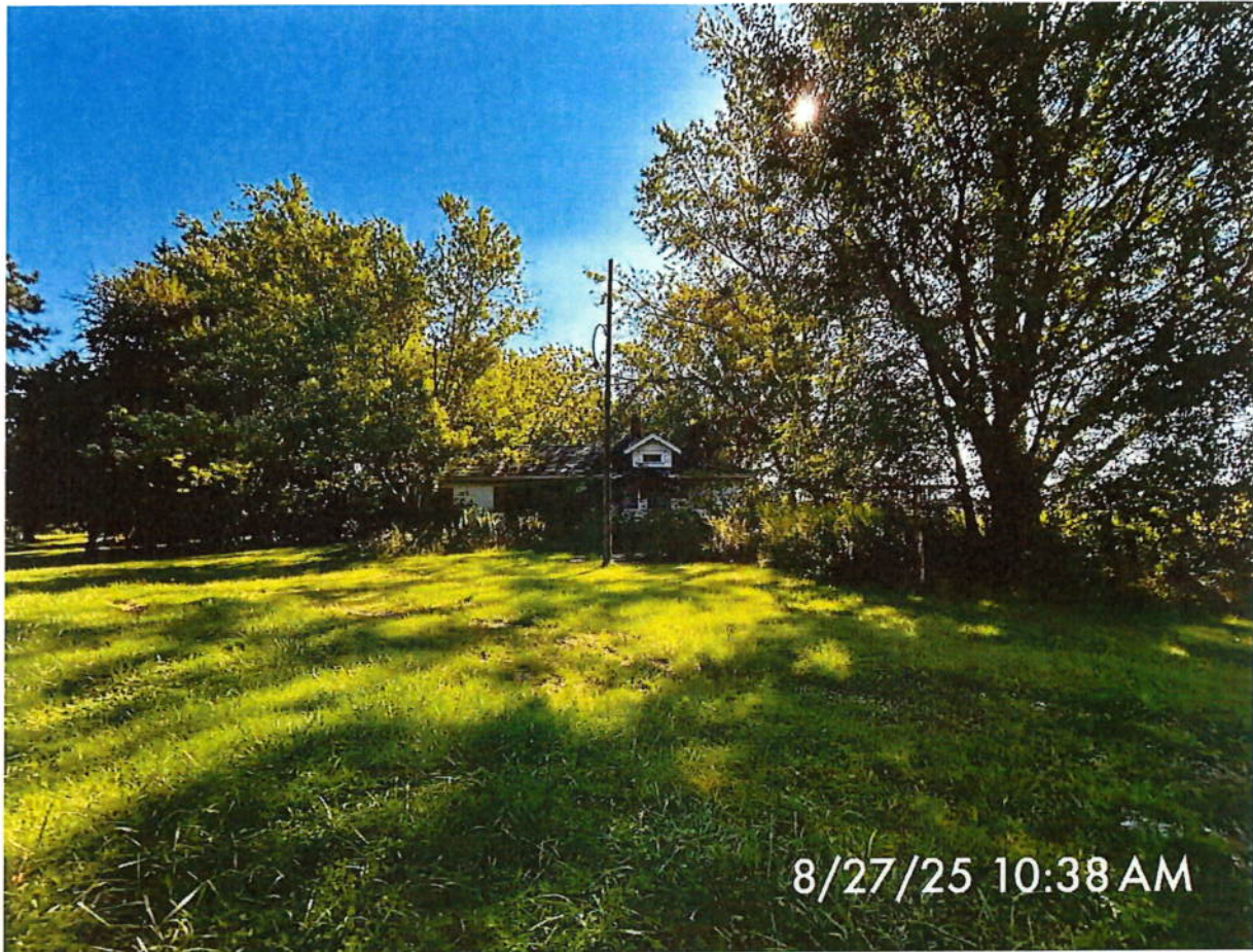
P5. Looking north toward the property and existing fire damaged house at 3729 Bremen Highway.
