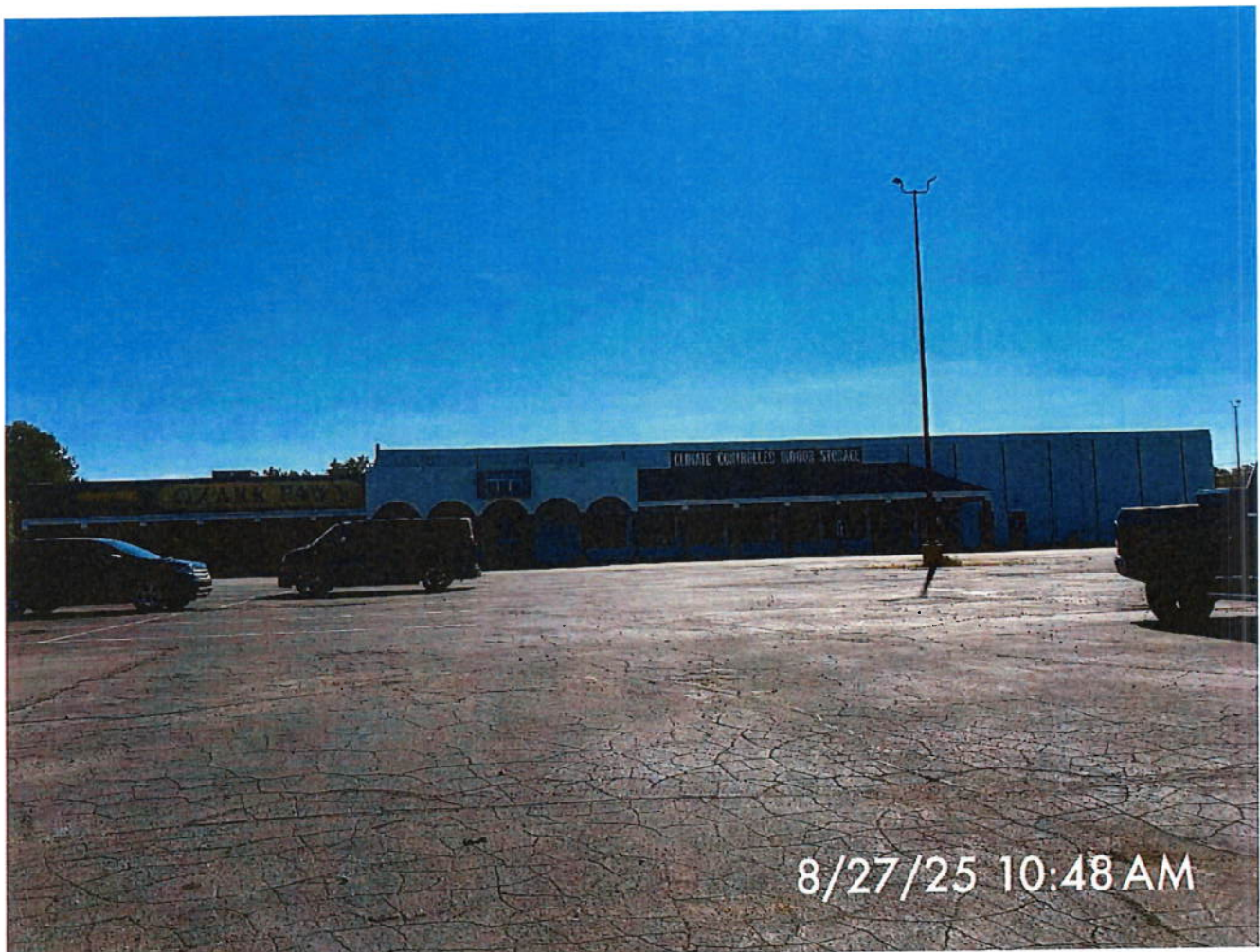
P1. Looking easterly from the subject property (parking lot) toward the multi-tenant commercial building.
