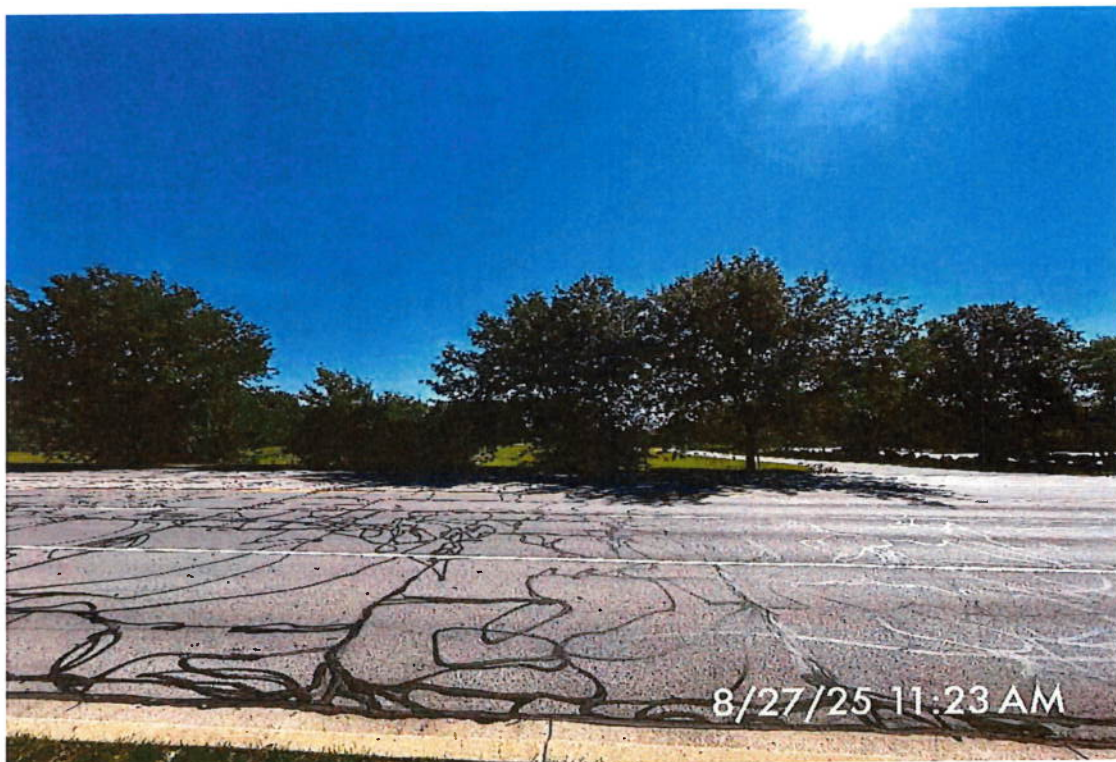
P1. Looking east toward vacant land from N Main Street
