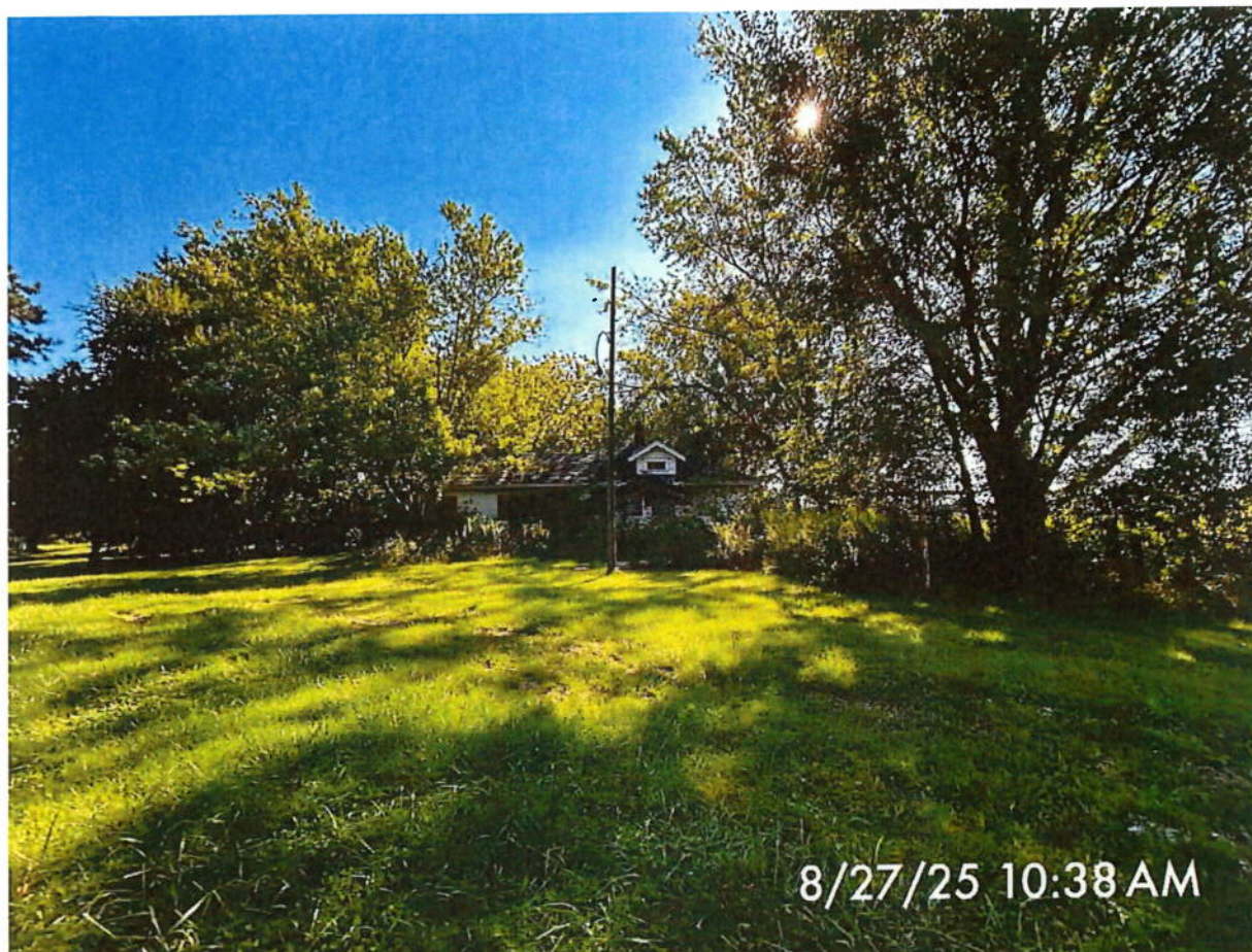
P5. Looking north toward the property and existing fire damaged house at 3729 Bremen Highway.
