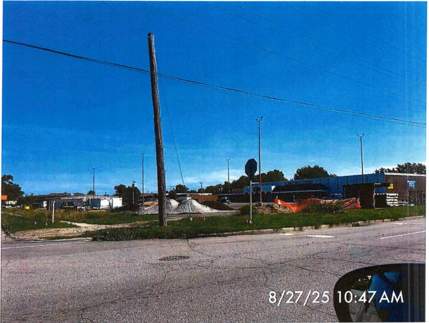
P2. Looking northeasterly from the S. Merrifield Ave. & E. 12 th St. intersection toward the property and multi-tenant commercial building to the east.
