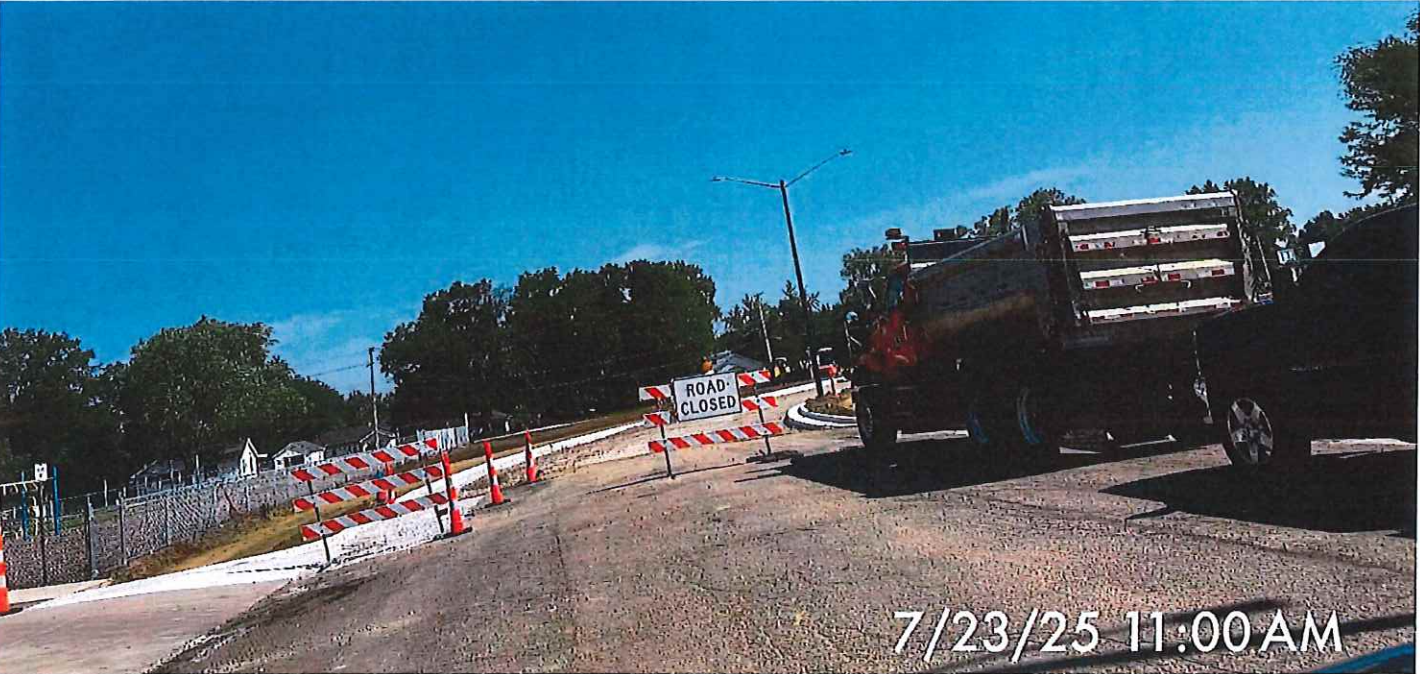
Ballard Street Road Construction
