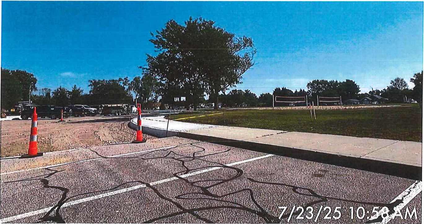
New Ballard Street from Twin Branch Park side
