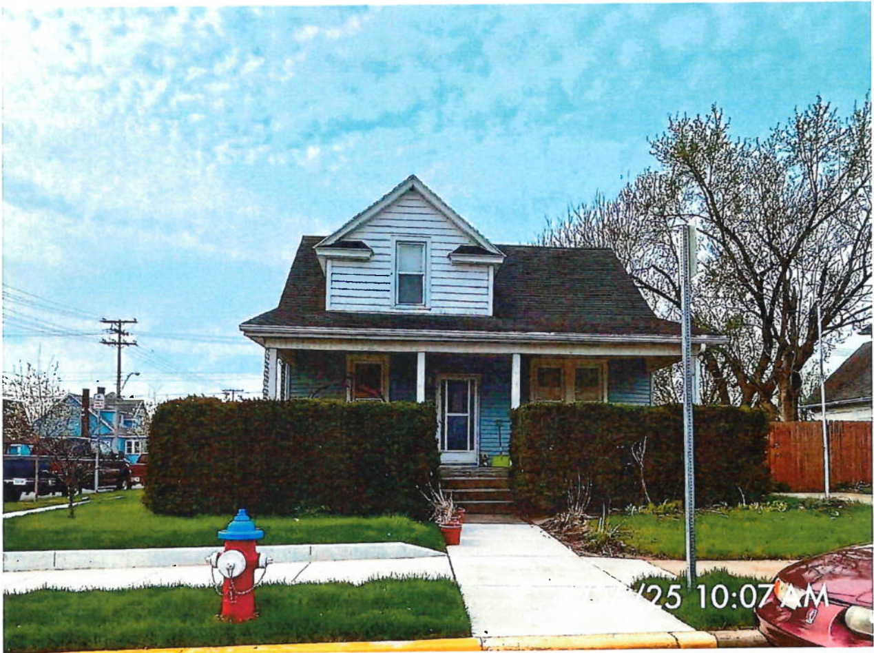
South facing from West Sixth Street
