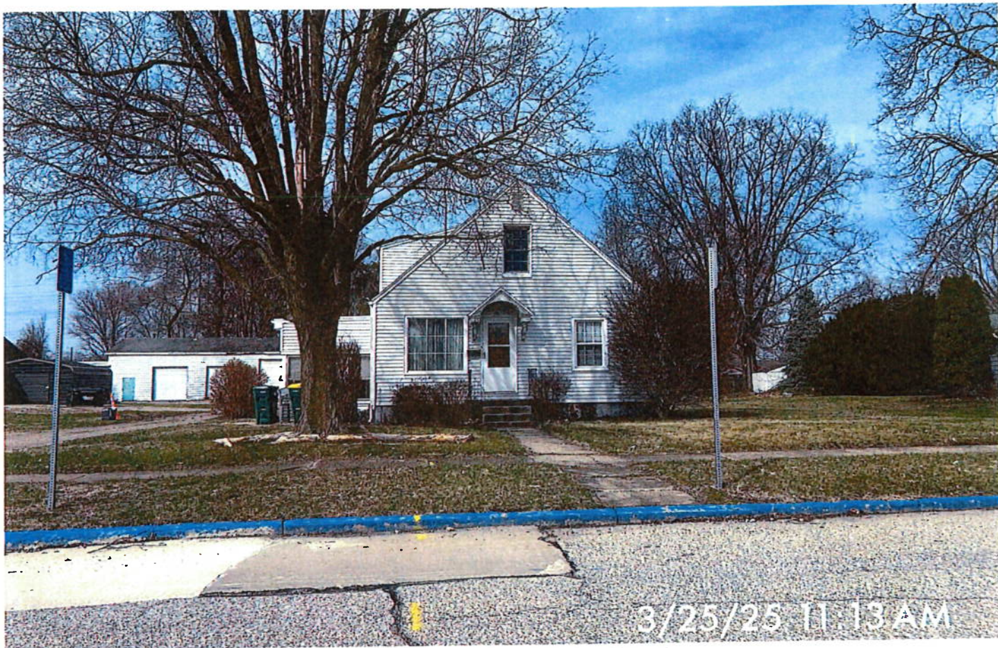
P1. Facing west from Virginia Street
