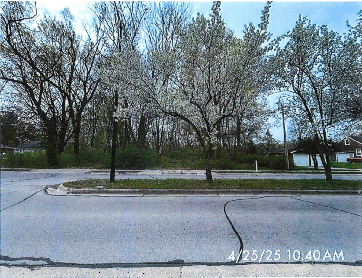
South facing from West Catalpa Drive
