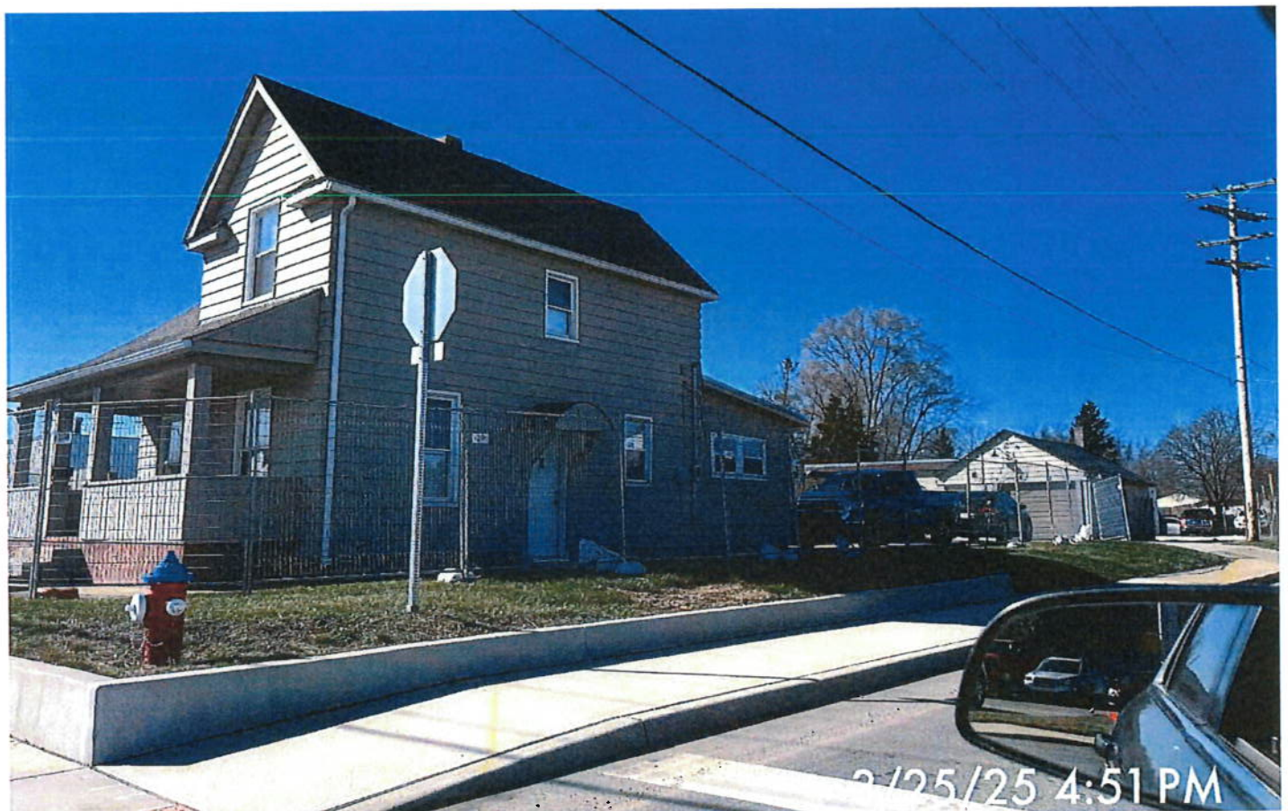
P4. Looking northwest from N Merrifield toward 1032 E Jefferson
