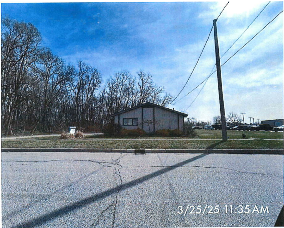
P1. Existing building at 2406 Schumacher (to be demolished). East facing from Schumacher Dr.
