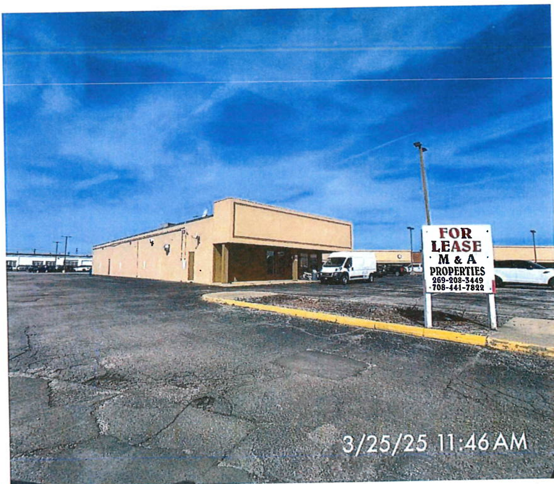
Northwest facing from the parking lot.
