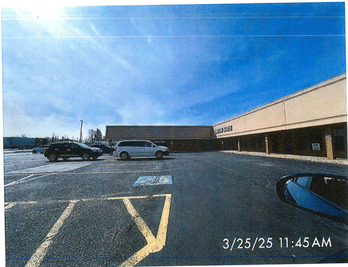
South facing from the parking lot.
