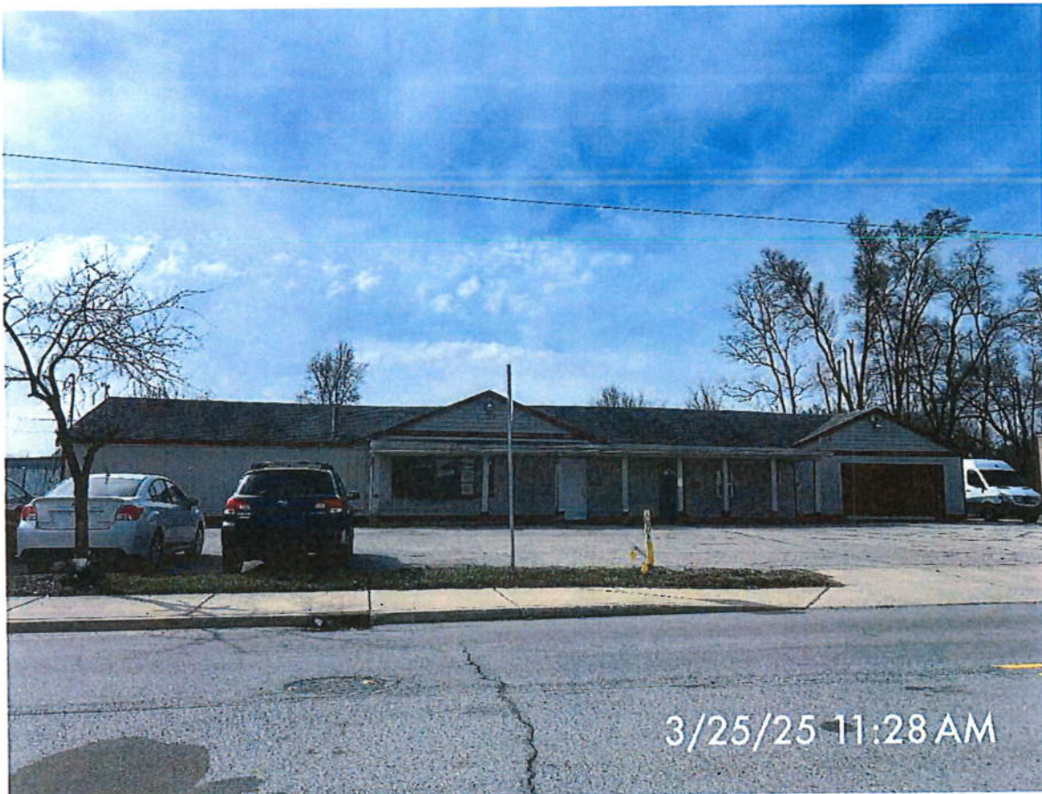
P2. Looking south from E Jefferson toward 1023 E Jefferson
