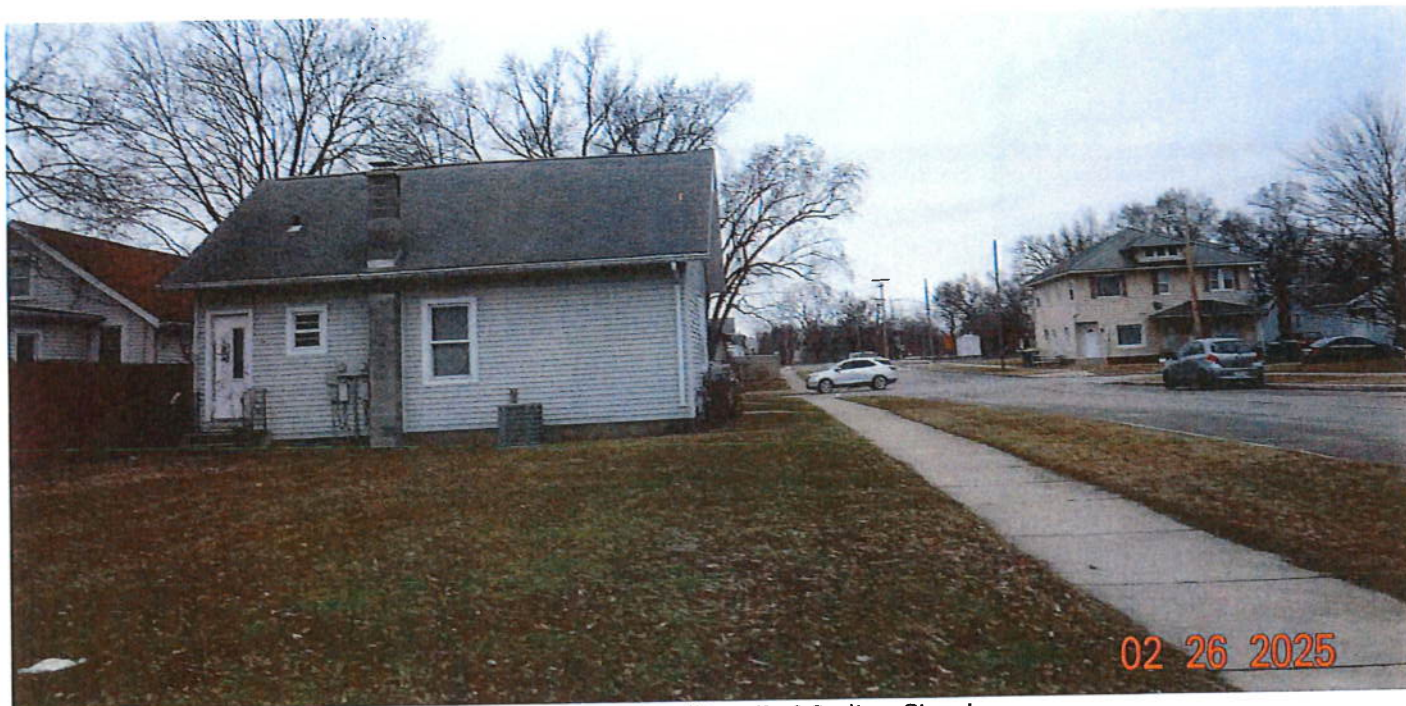
Facing north from alley off of Carlton Street
