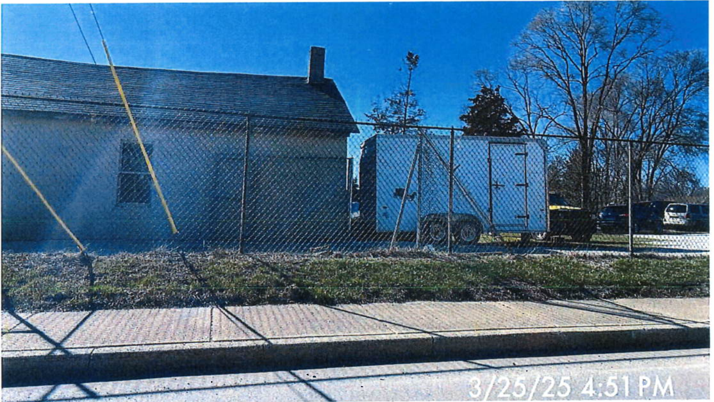
P5. Looking west from N Merrifield toward rear of 1032 E Jefferson
