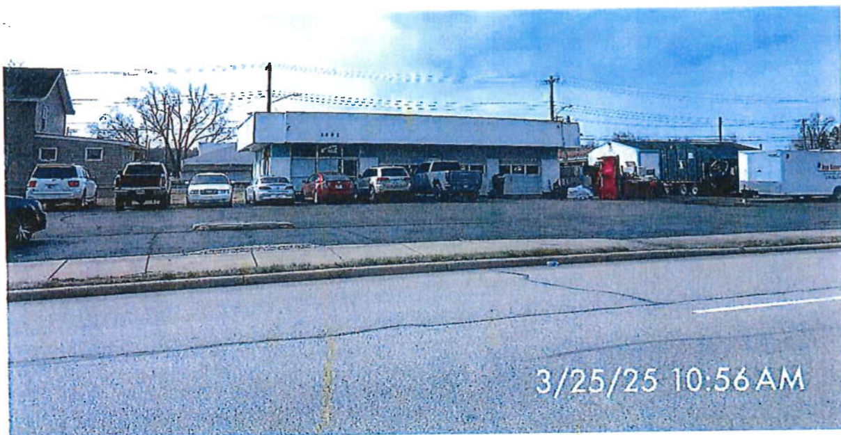
Site looking south from Lincolnway West
