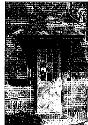
Fig. 16 South entry door
