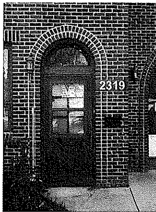
Fig. 4 North entry door
