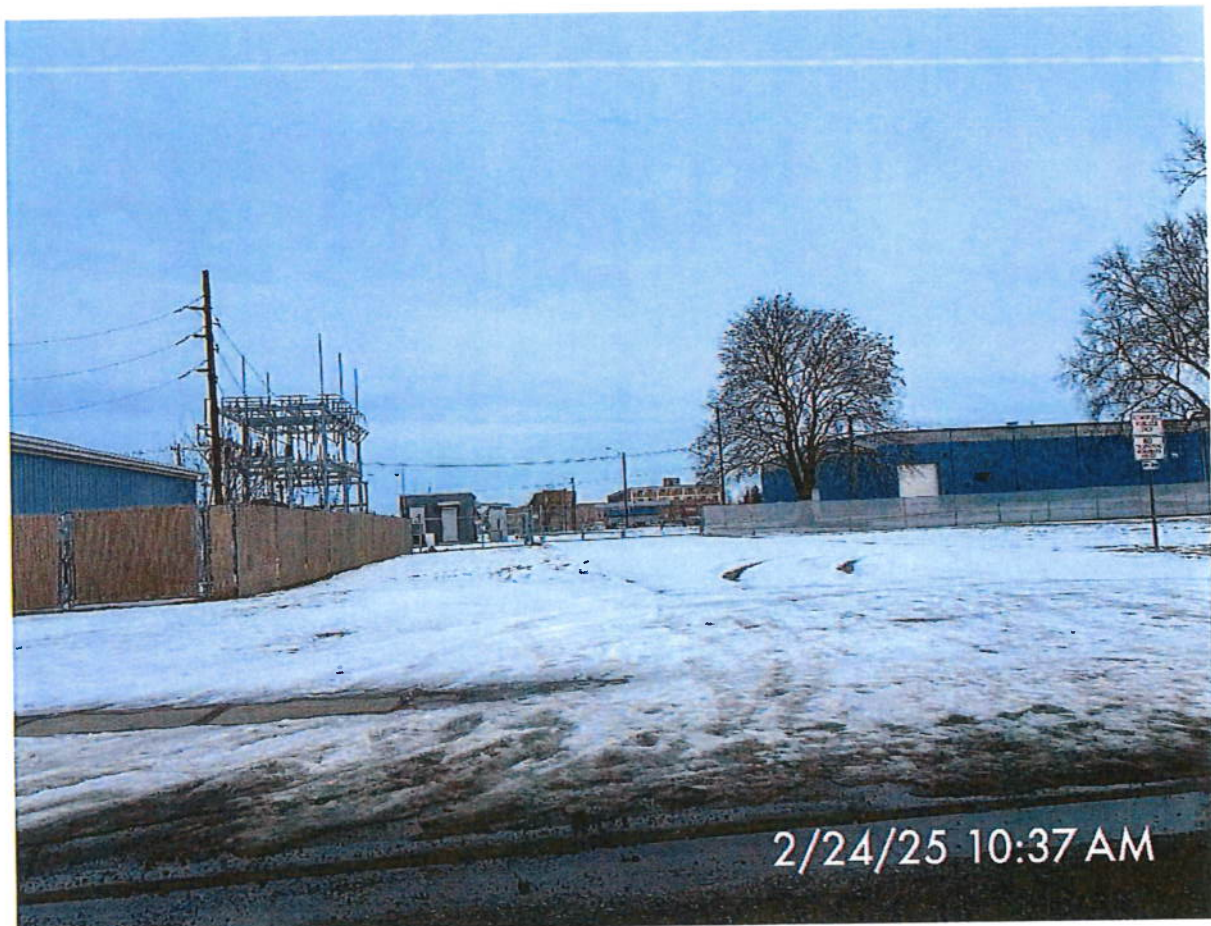
North facing from East Tenth Street
