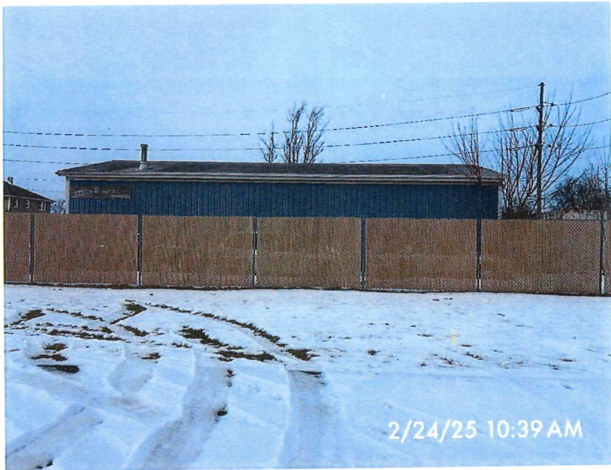
West facing from the access drive
