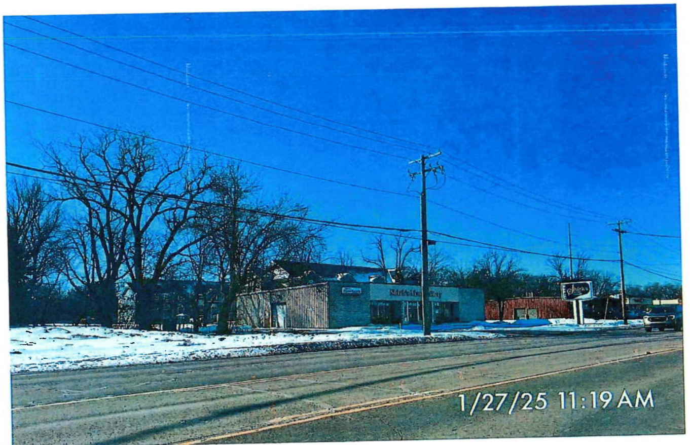
Southwest facing from West Edison Road
