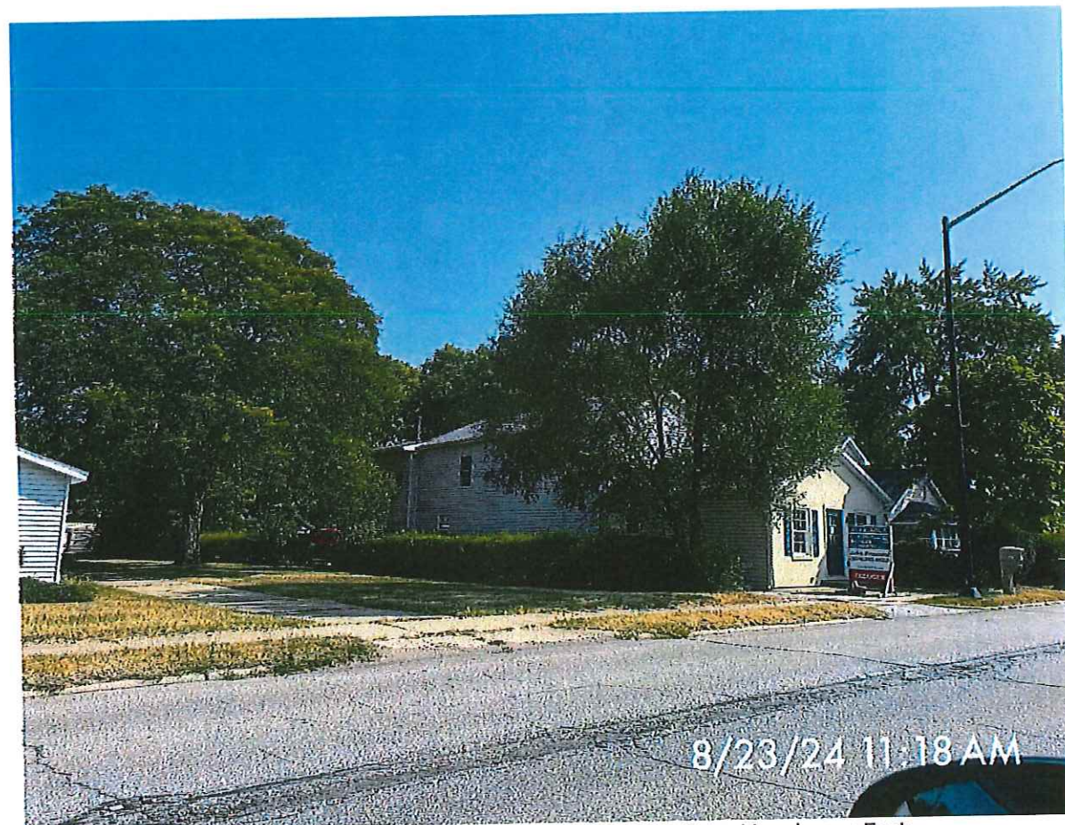
P1. Looking northwesterly toward the property from Lincolnway East.
