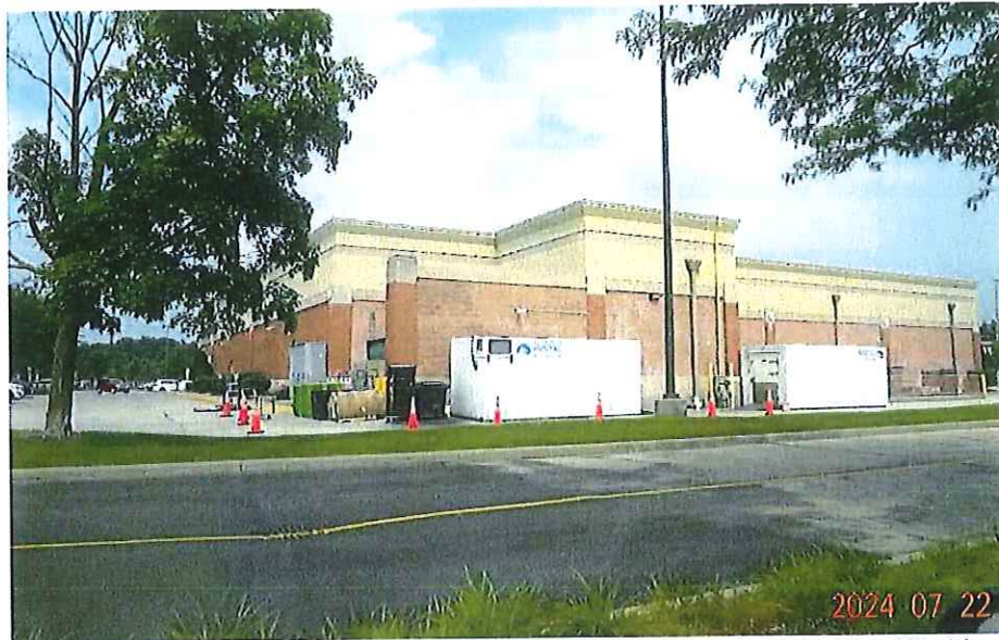
A view of the storage containers from the access drive into Princess City Plaza
