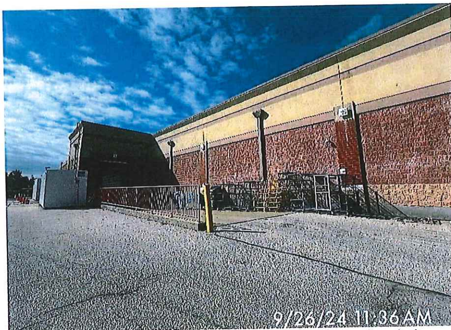
A view of additional outside storage, racks, in the loading dock.
