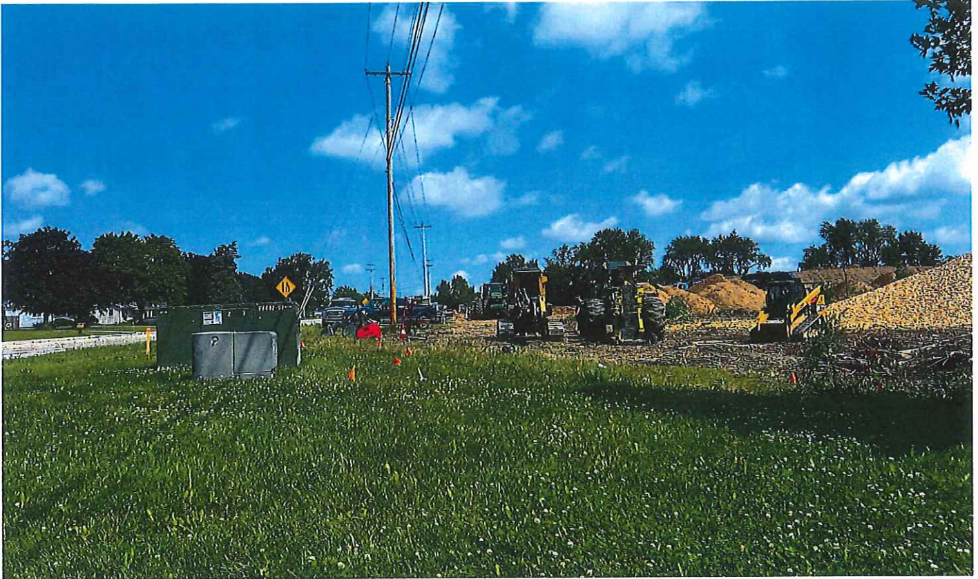
P1 North facing from corner of Beacon Parkway and Fir Road
