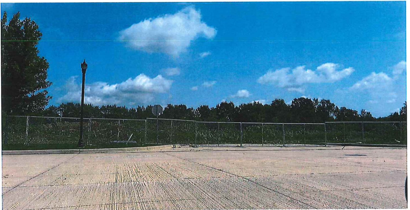
P2 North facing from Beacon Parkway
