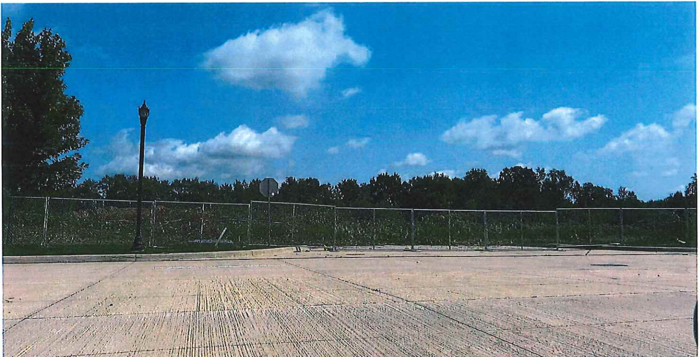
P2 North facing from Beacon Parkway
