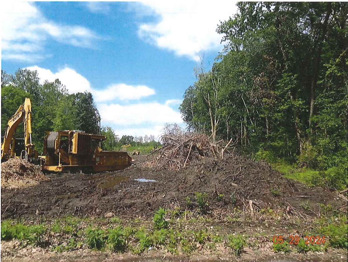
P5. Looking west from Clover Road toward the southeast corner of the property.
