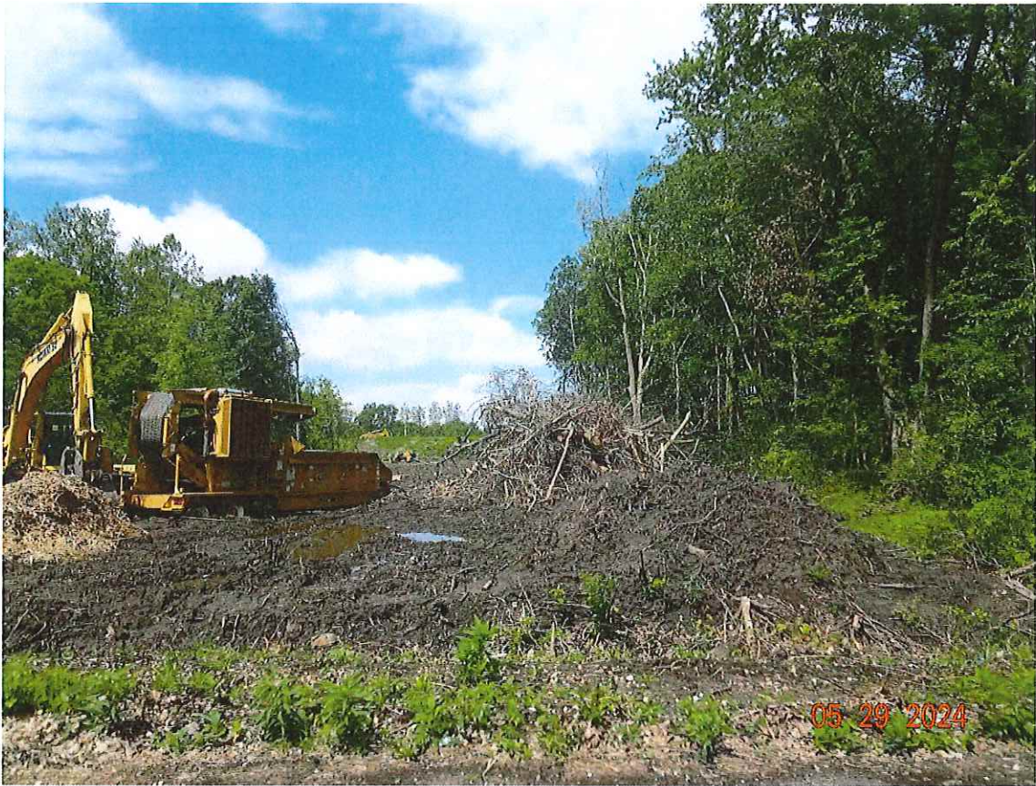
Looking west from Clover Road toward the southeast corner of the property.
