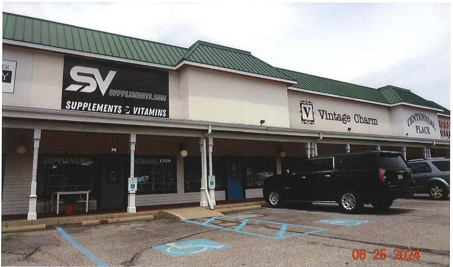
Northeast facing from the parking lot
