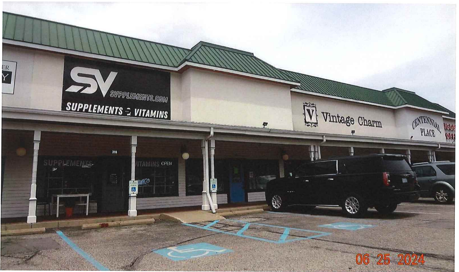
Northeast facing from the parking lot
