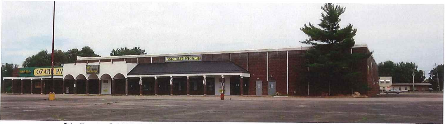
P1. Front of 1010 S. Merrifield, operating as MCC Self Storage (facing west)
