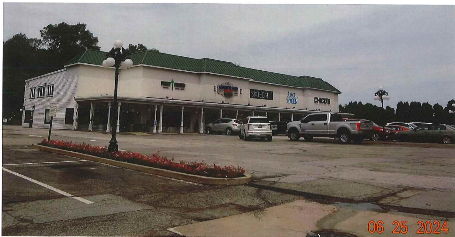
Northeast facing from the parking lot
