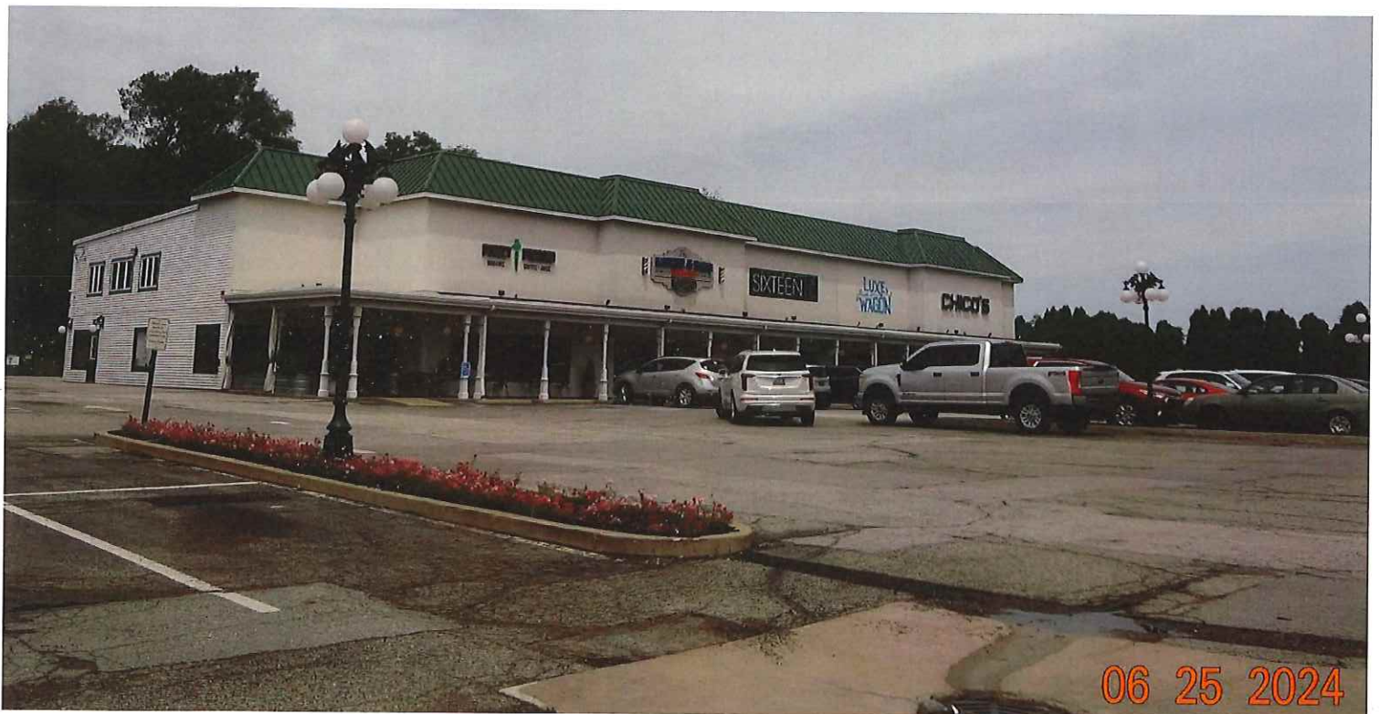
Northeast facing form the parking lot
