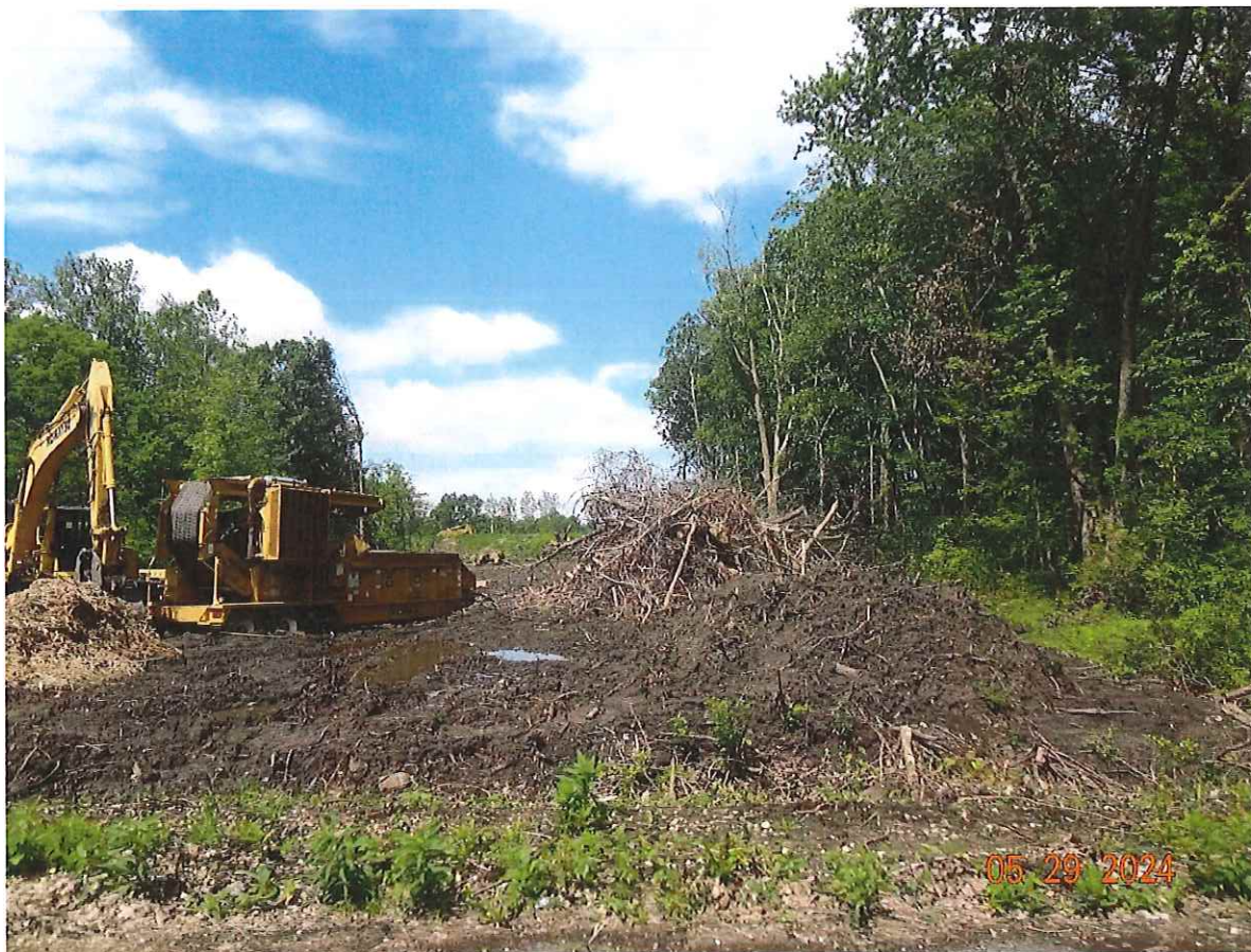
P5. Looking west from Clover Road toward the southeast corner of the property.
