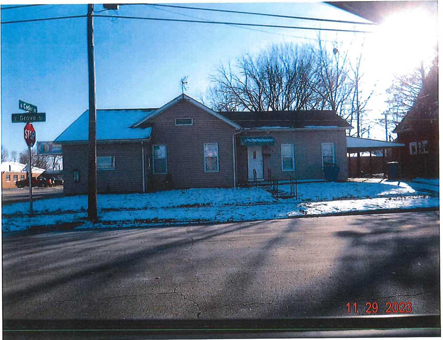
617 E Grove Street – looking south from E Grove Street
