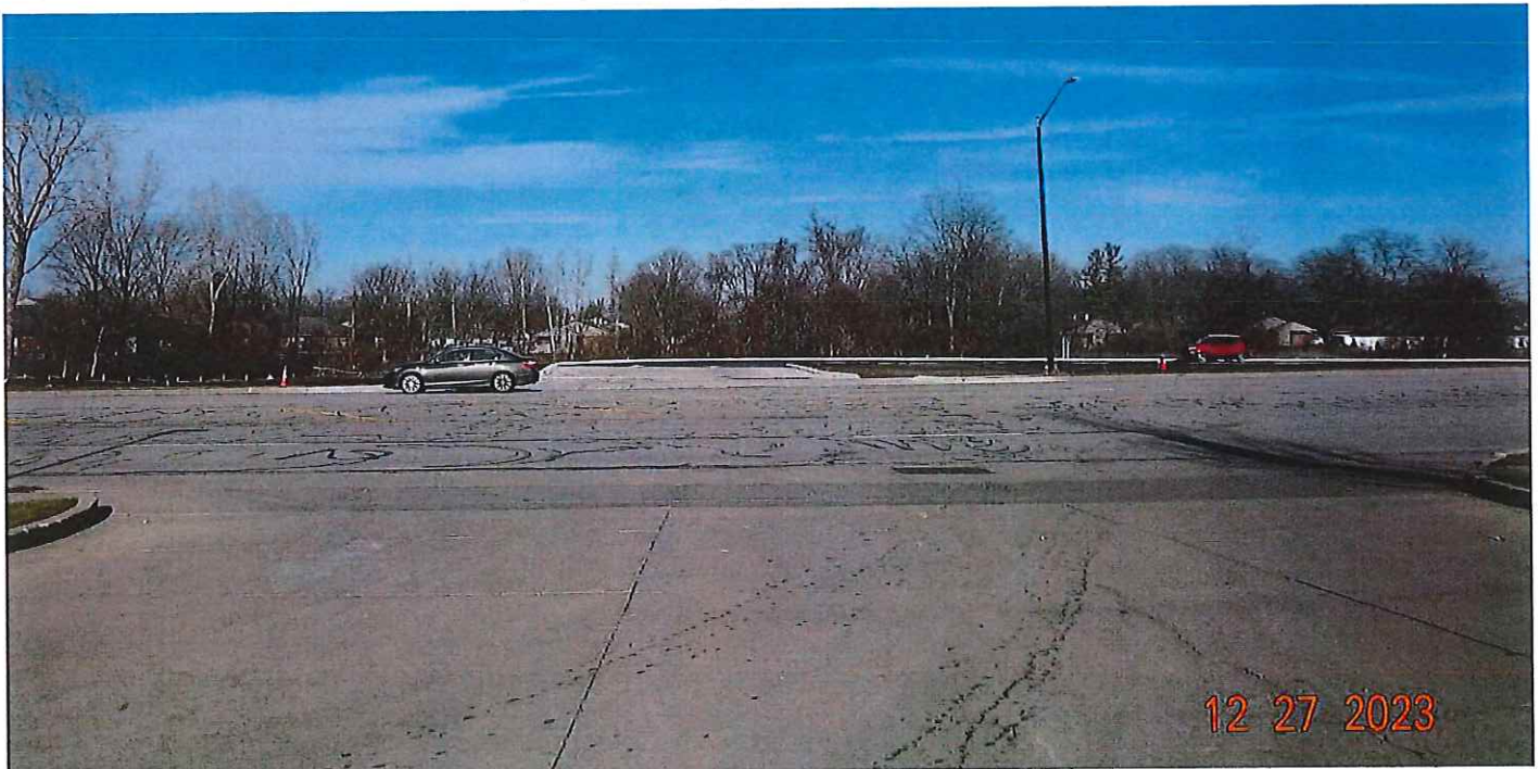
P1. Looking north toward the property from the eastern Charlie's Phillips 66 access drive on the south side of E. 12 th St. at the newly installed access drive
