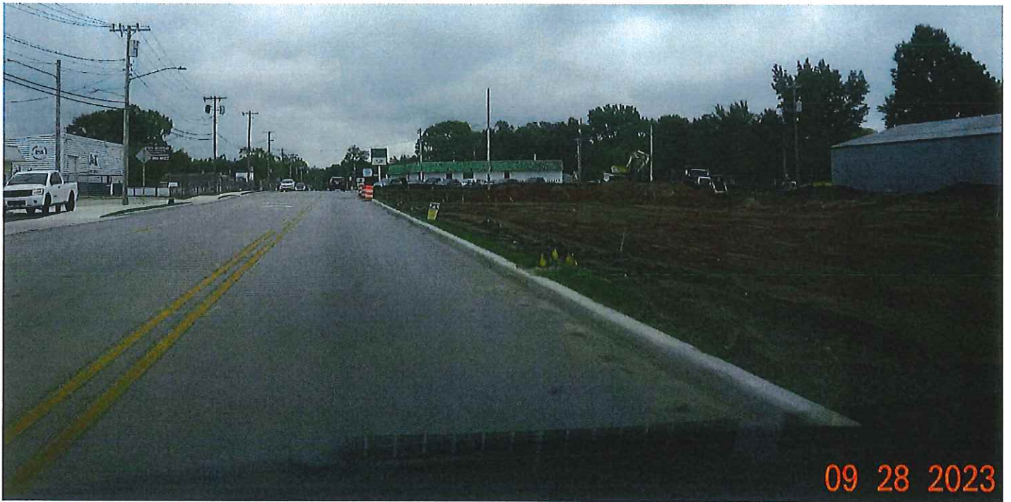
P1. A view of the Reggio's property from the intersection of Jefferson and Merrifield (showing construction).
