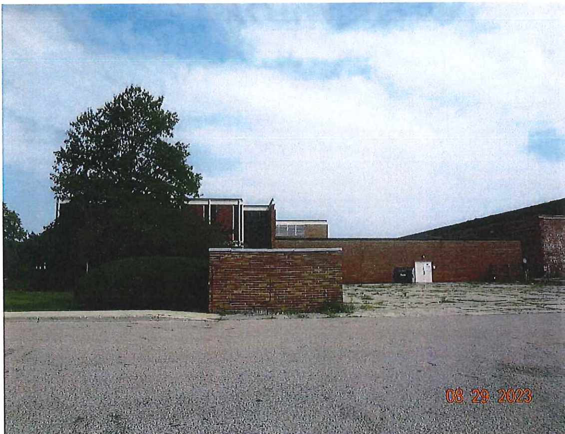
P5. Loading dock area on south side
