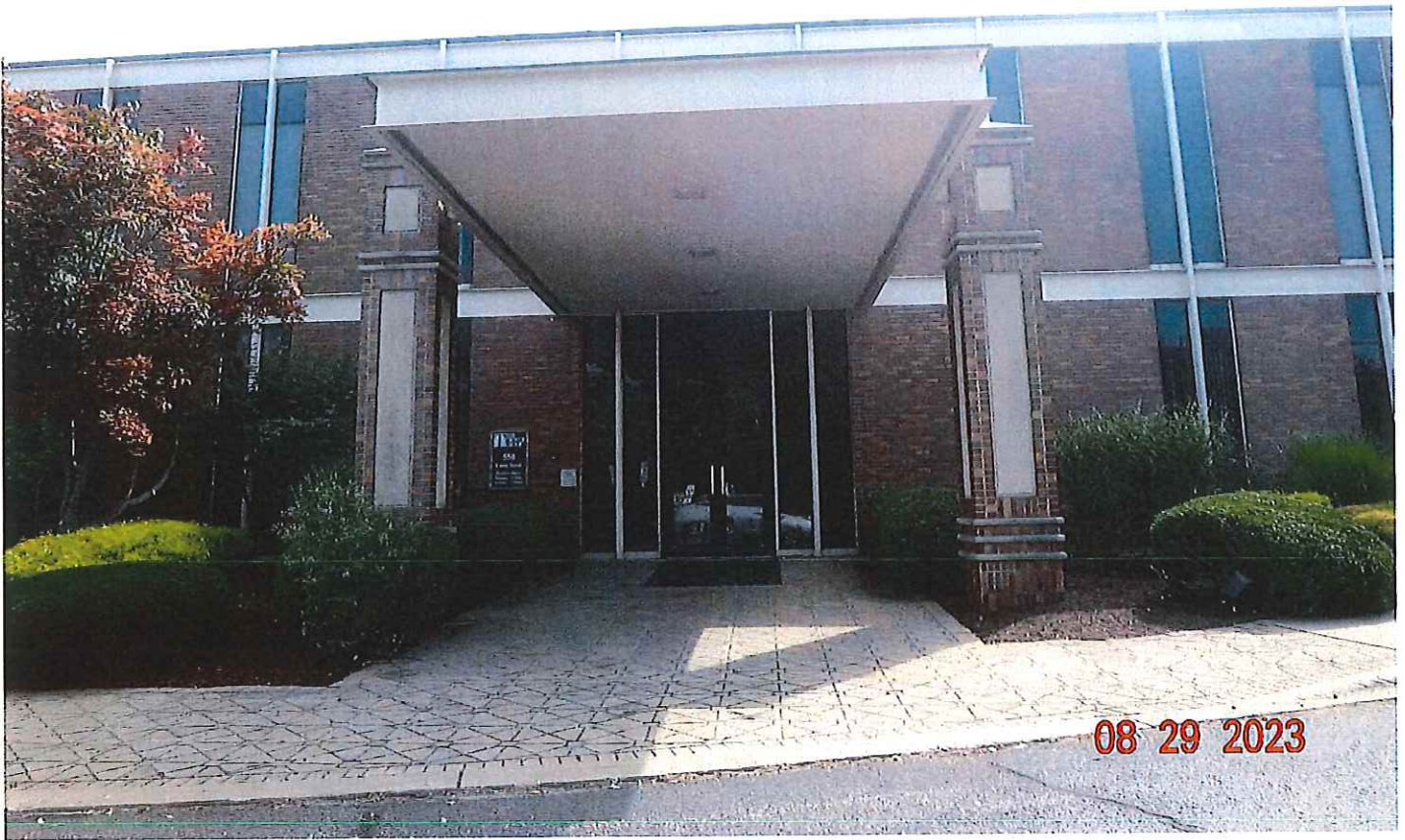
P3. Front entrance facing Union Street
