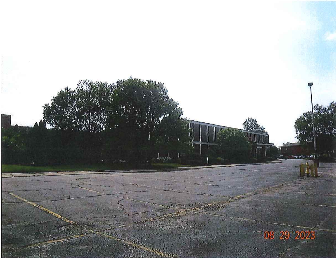
P4. Looking south from parking lot.
