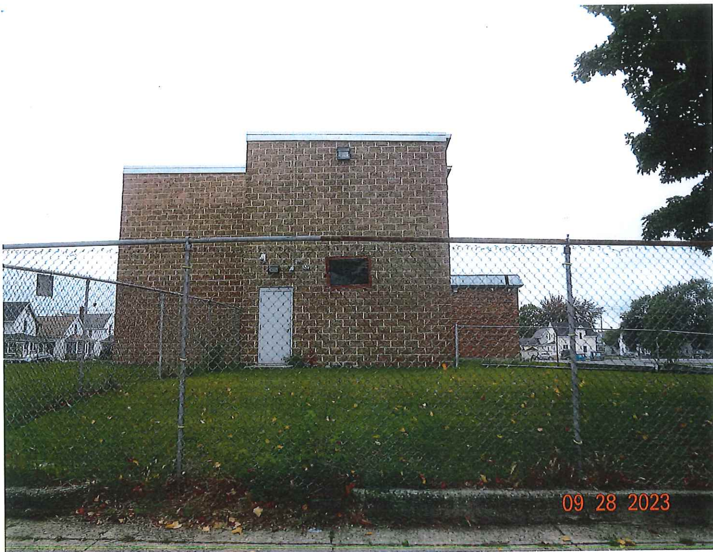
P4 West facing from South Mill Street
