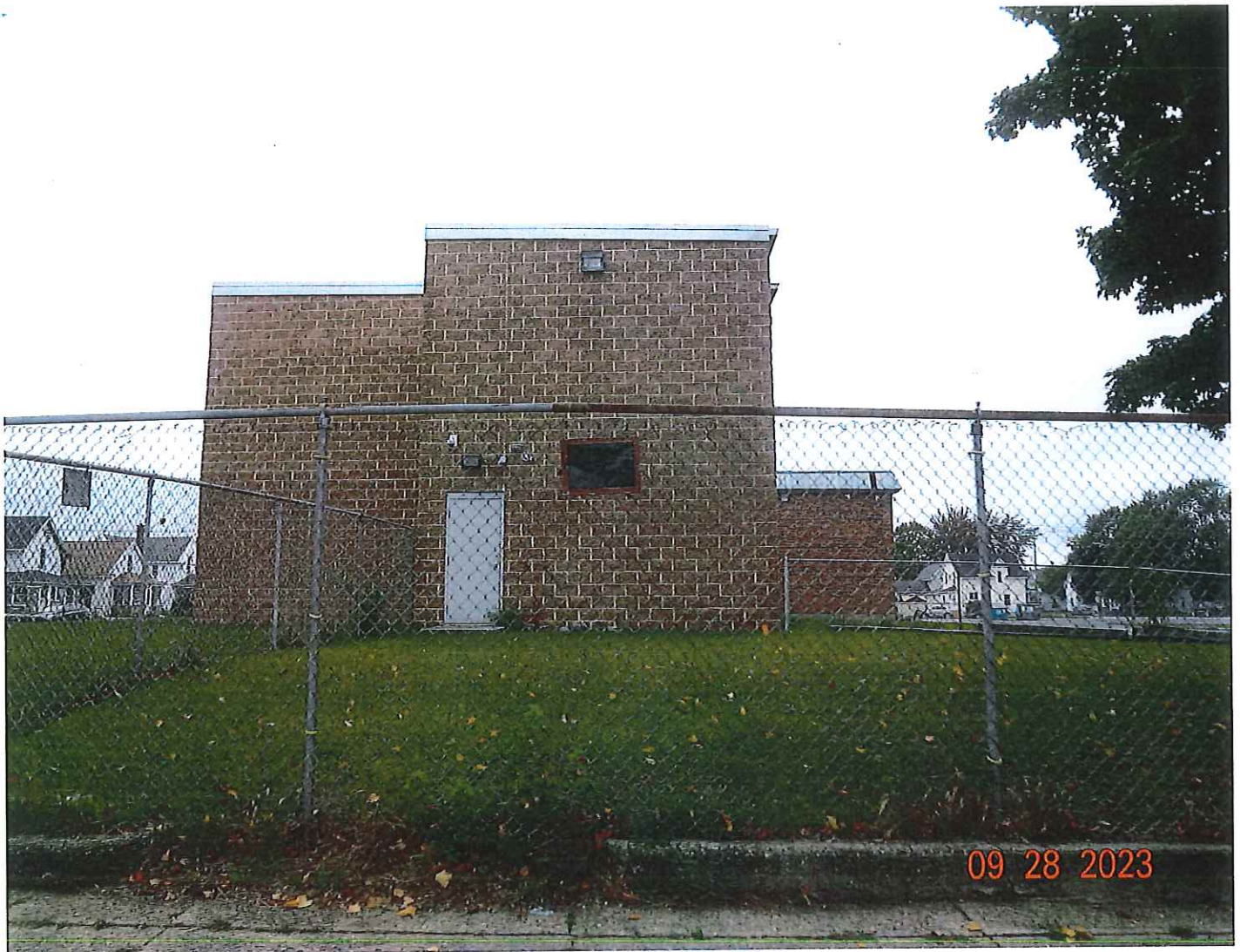
P4 West facing from South Mill Street
