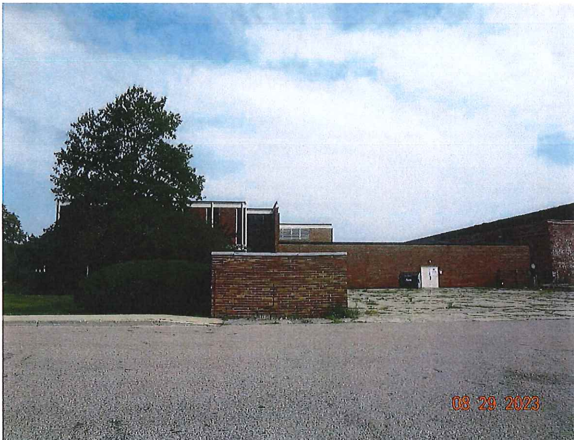
P5. Loading dock area on south side
