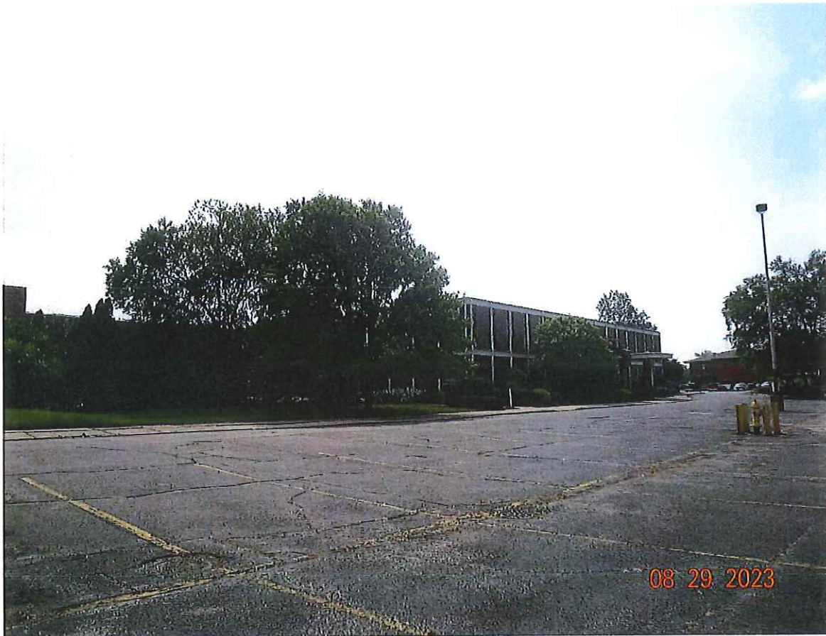
P4. Looking south from parking lot.
