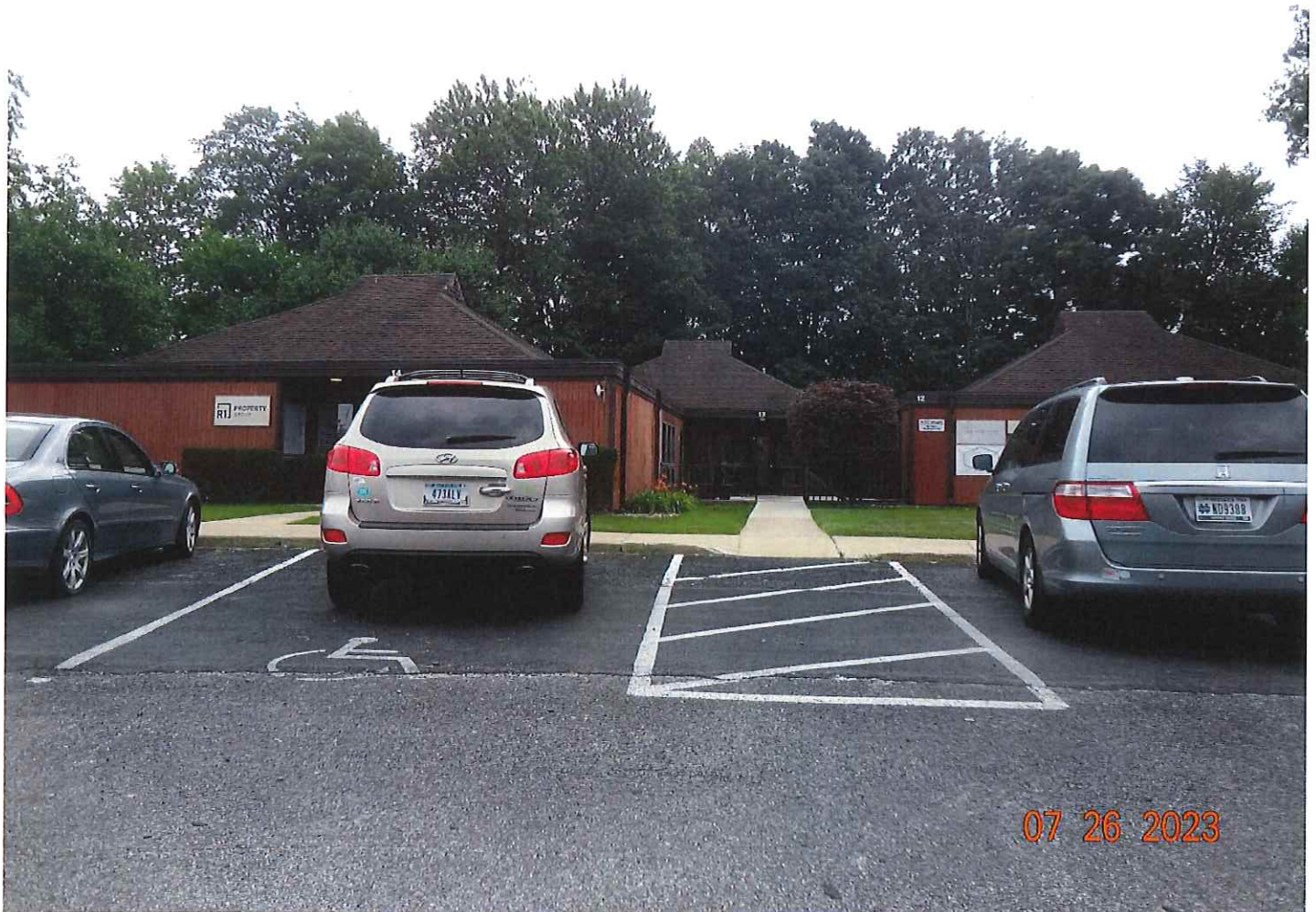
Front view of Unit 14 and adjacent units
