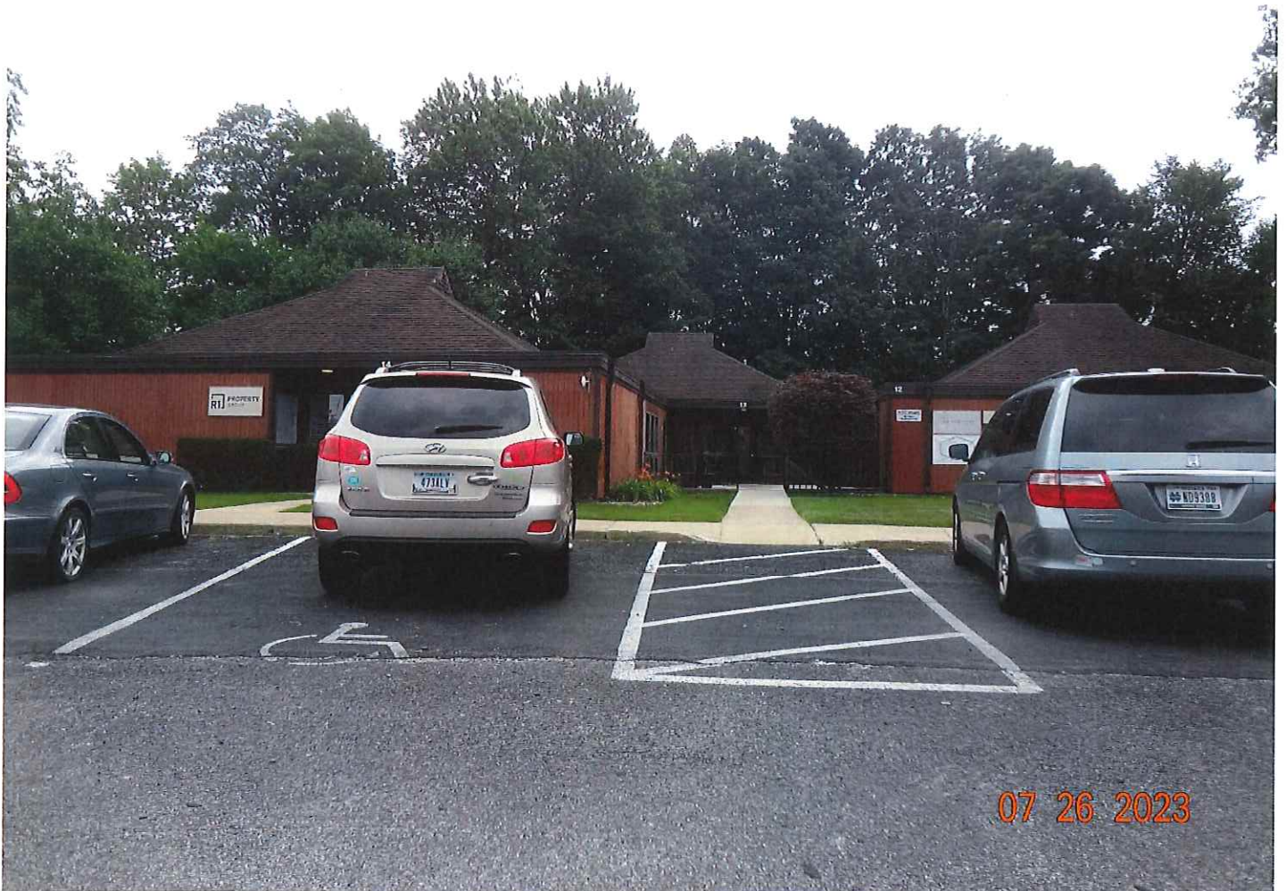
Front view of Unit 14 and adjacent units
