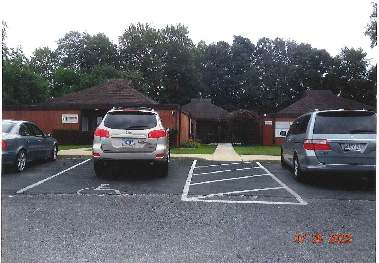
Front view of Unit 14 and adjacent units
