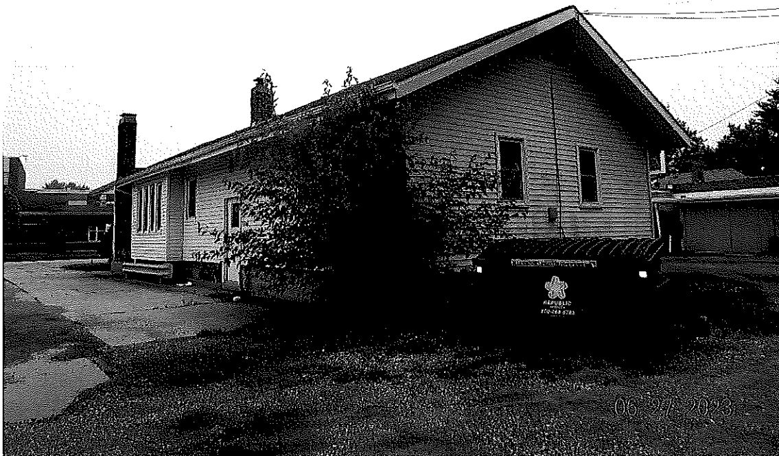
A view of the parking lot and rear of building from the East
