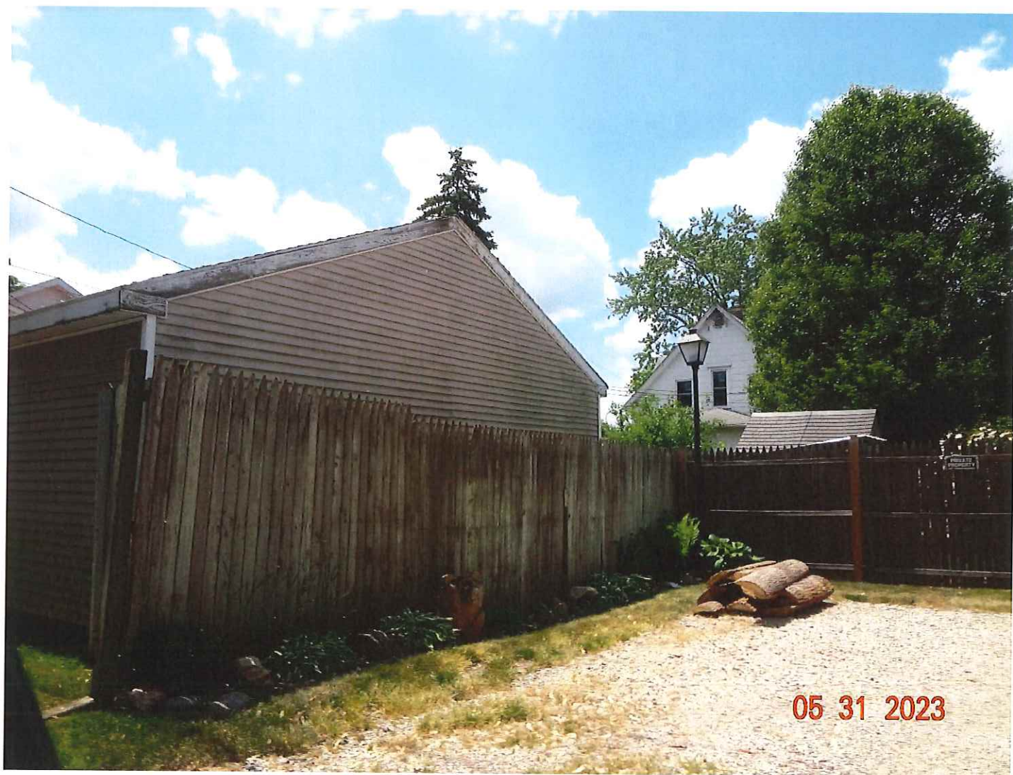
Rear view of 712 Division Street (white house in background)
