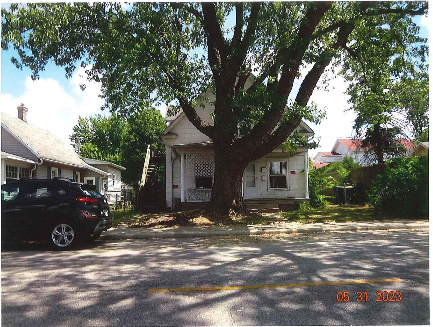
Front view of 712 Division Street
