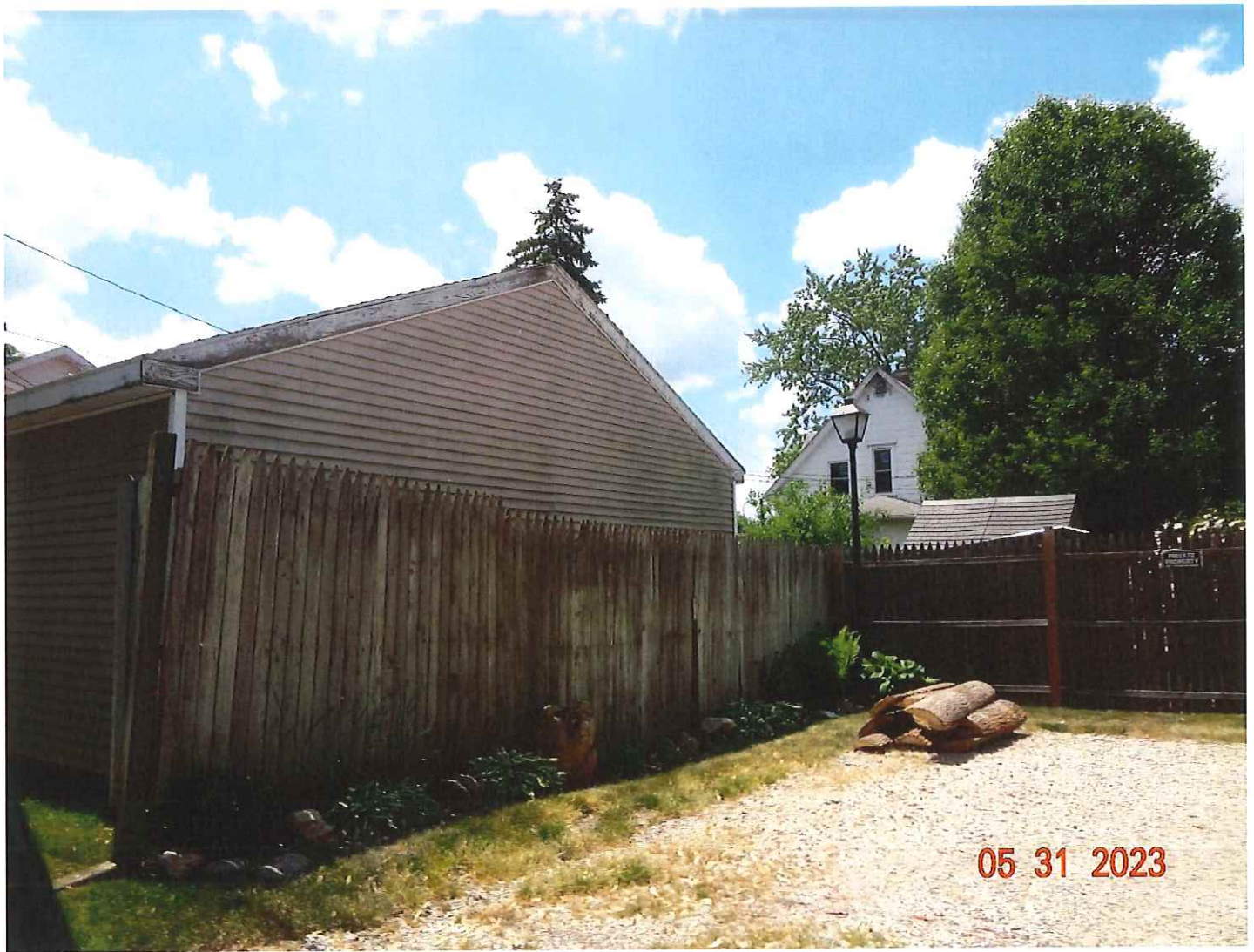
Rear view of 712 Division Street (white house in background)
