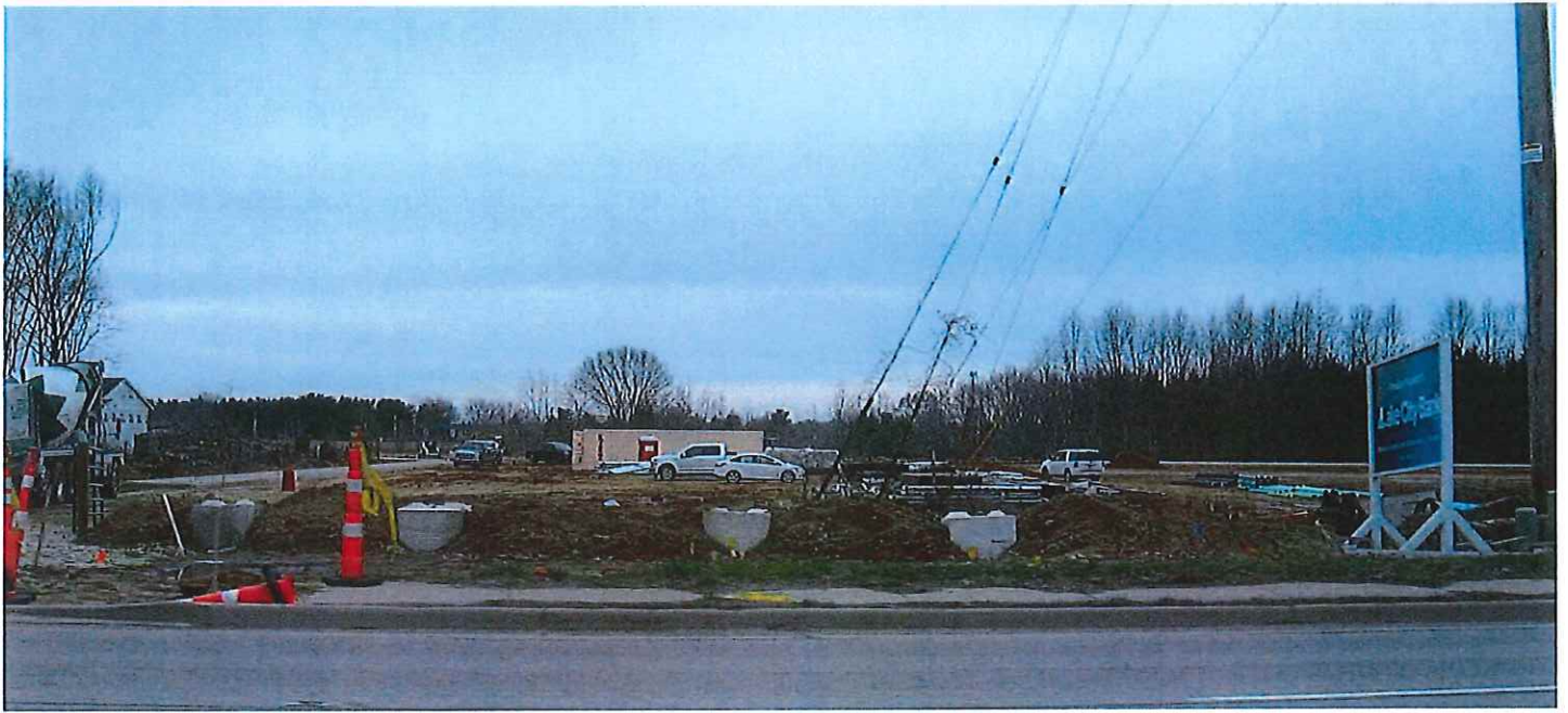
P3. Storage units to the north under construction.
