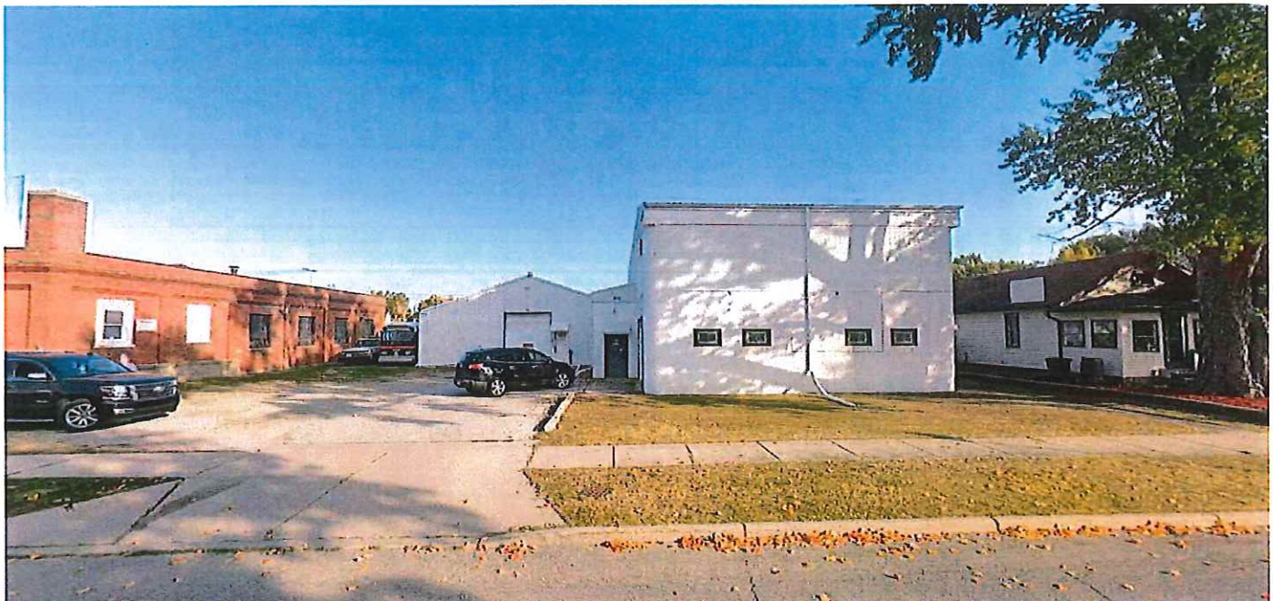
North facing from W Sixth St
