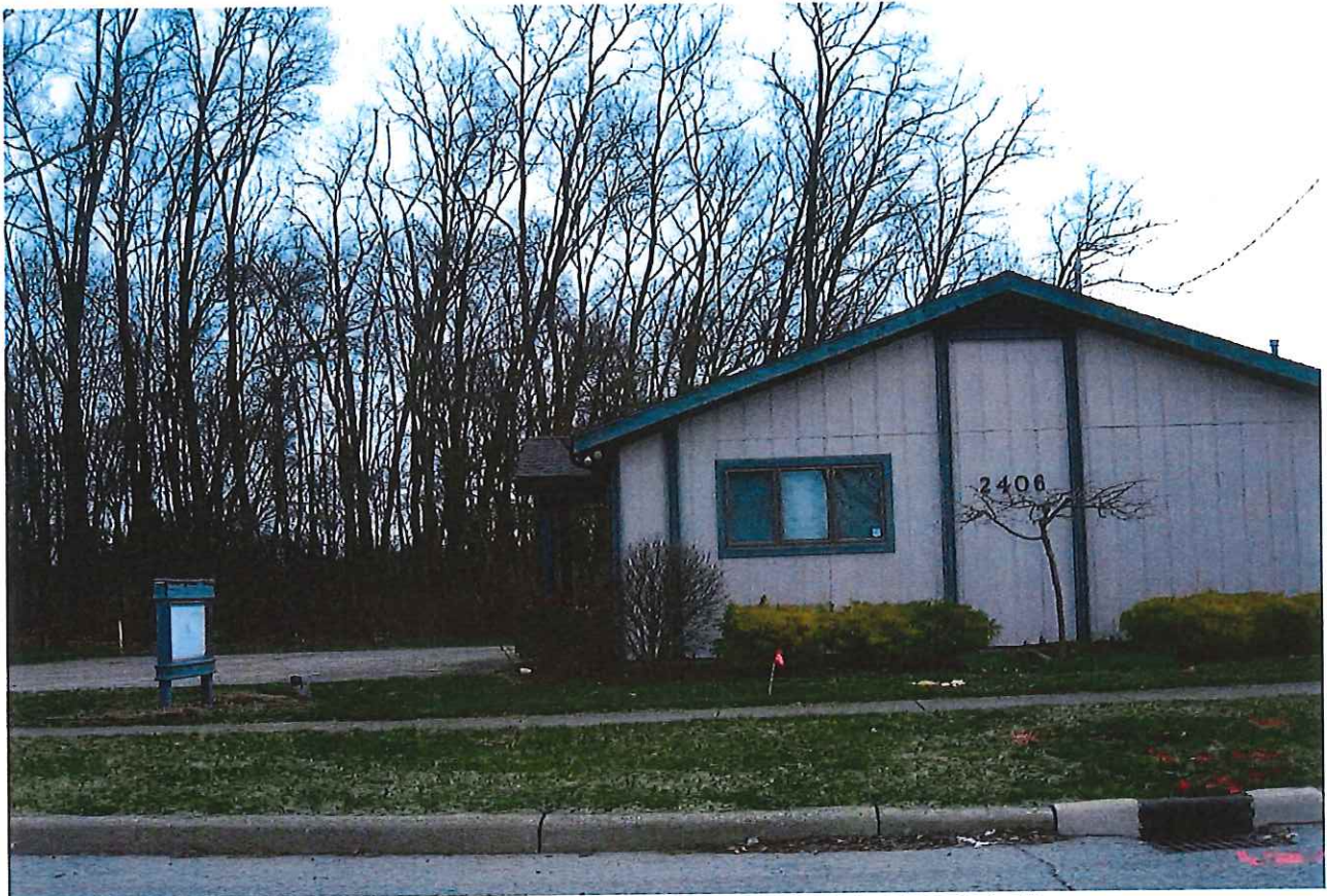
P1. Existing building at 2406 Schumacher (to be demolished)
