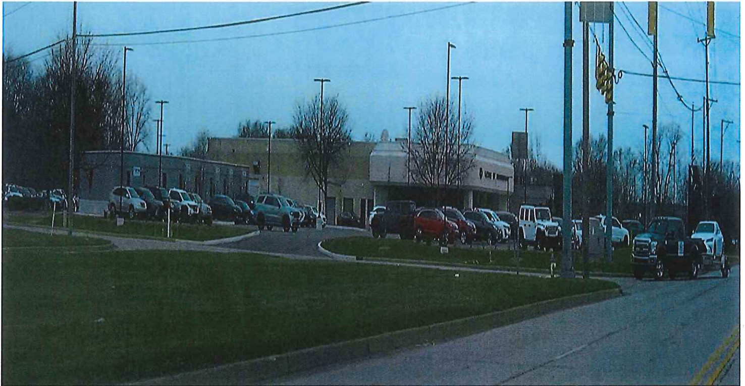
Northwest facing from Grape Road
