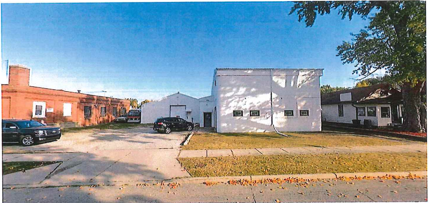
North facing from W Sixth St
